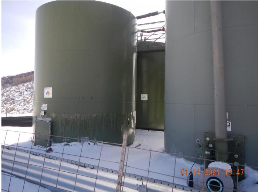
**Capacity on production tank is too small to be seen from a distance.**
