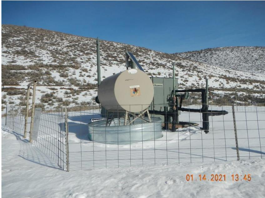
**Label on methanol tank is damaged and tearing.**
