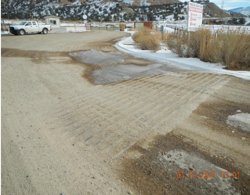
Tracking cattle guard is packed with sediment at main gate.
