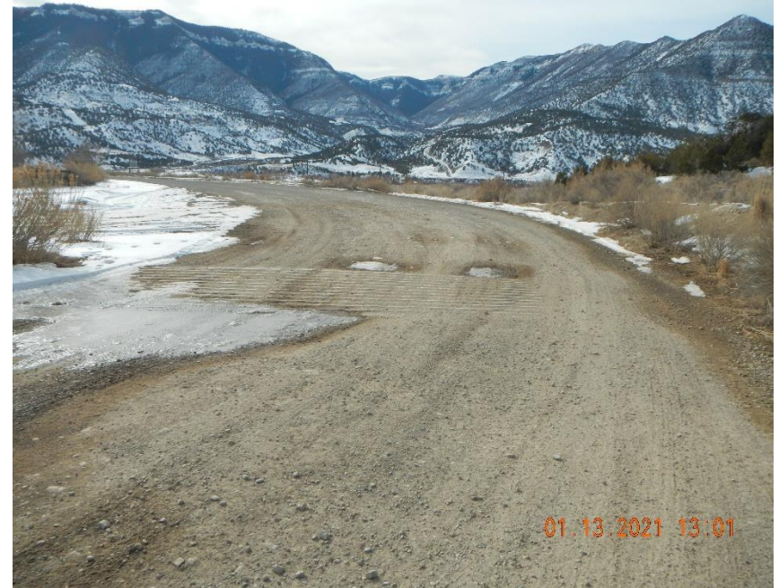
Tracking cattle guard is packed with sediment at main gate.
