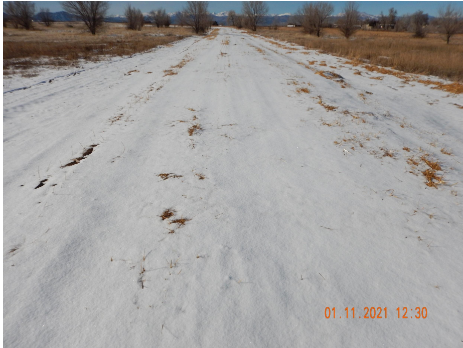
Photo 1. Photo taken from the entrance of the location off Hwy 287, facing West. Photo illustrates the Operator has performed final reclamation activities with the evidence of straw crimped mulch.
