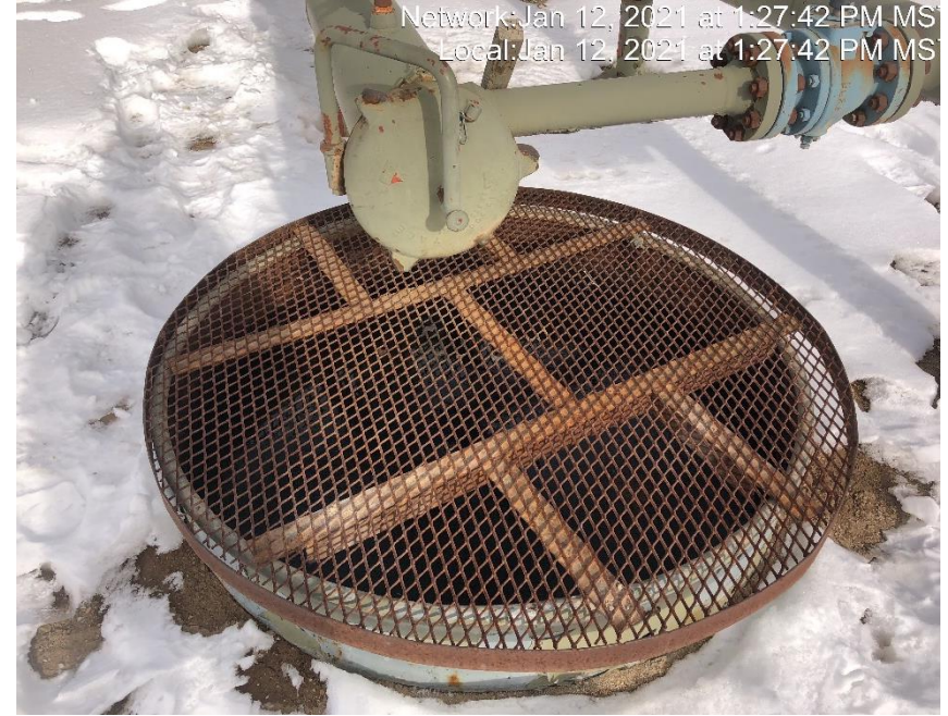
Photo #2620 Oily fluids in pig station containment.
