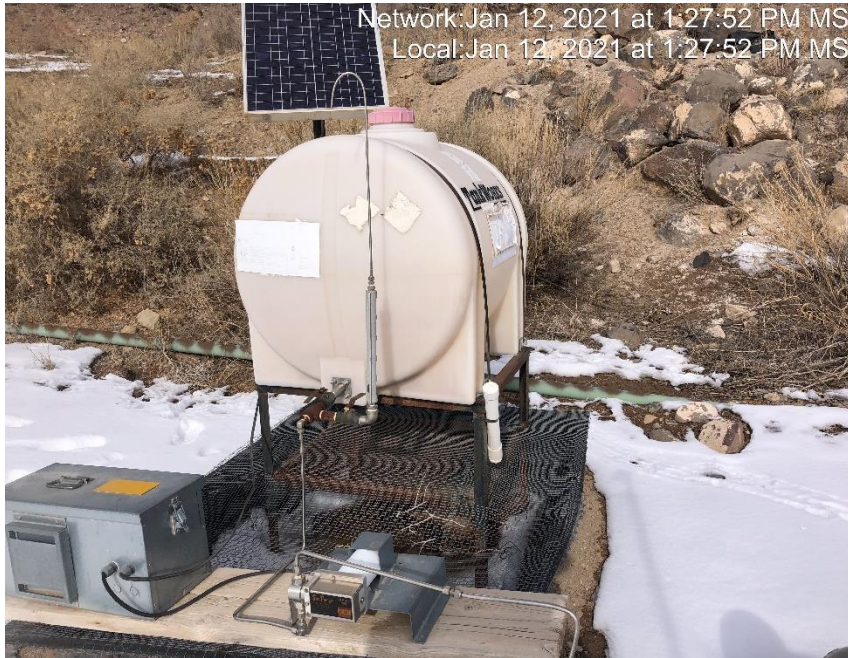
Photo #2621 Chemical tank label weathered and not legible.
