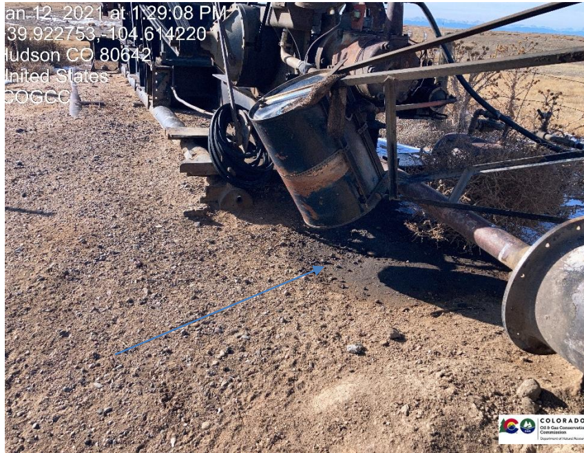
Pic 3 stained soil no BMP under chemical tank
