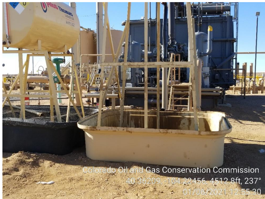
Photo 13 – Day Tank Containment Netting is in disrepair
