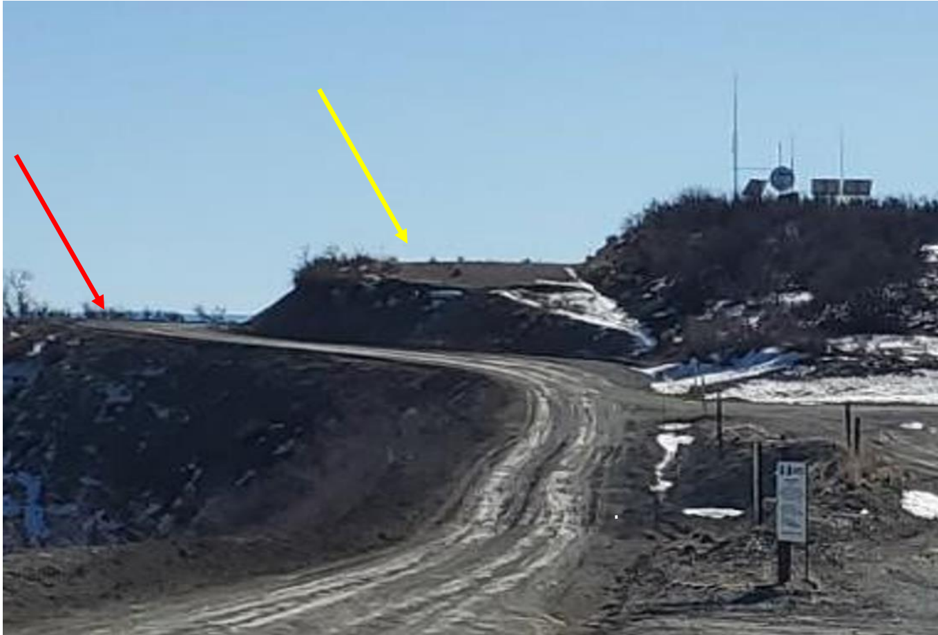
Photo 10: Continued from photo 9. Between 2011 and 2014, the access road in this area was further expanded to the east (red arrow). This photo shows that the original access road (yellow arrow) was not reclaimed; These areas will also require reclamation including, but not limited to, compaction alleviation, recontouring/regrading and revegetation.
