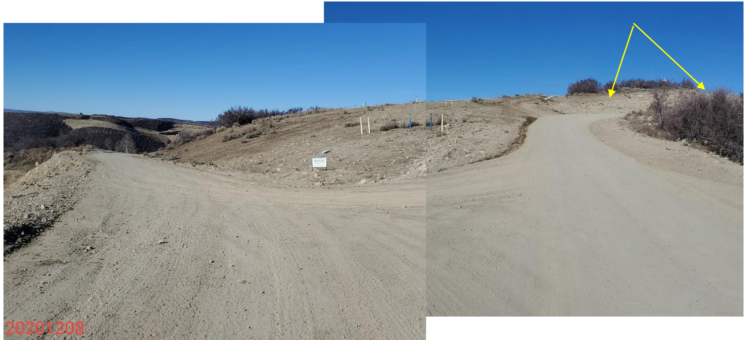
Photo 12: Photo taken from the south of the CC 0604-1 Pad Location, facing north. Photo shows the two access roads that run parallel to one another to the CC 0604-1 Pad. Photo also shows the section of the original access road (continued from photo 10, yellow arrows) that was not reclaimed when the access road was expanded further east between 2011 and 2014. These areas will also require reclamation including, but not limited to, compaction alleviation, recontouring/regrading and revegetation.
