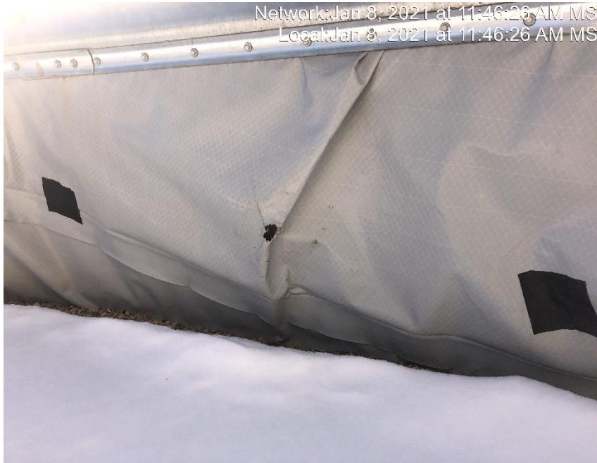
Photo #2584 Hole in tank containment liner.
