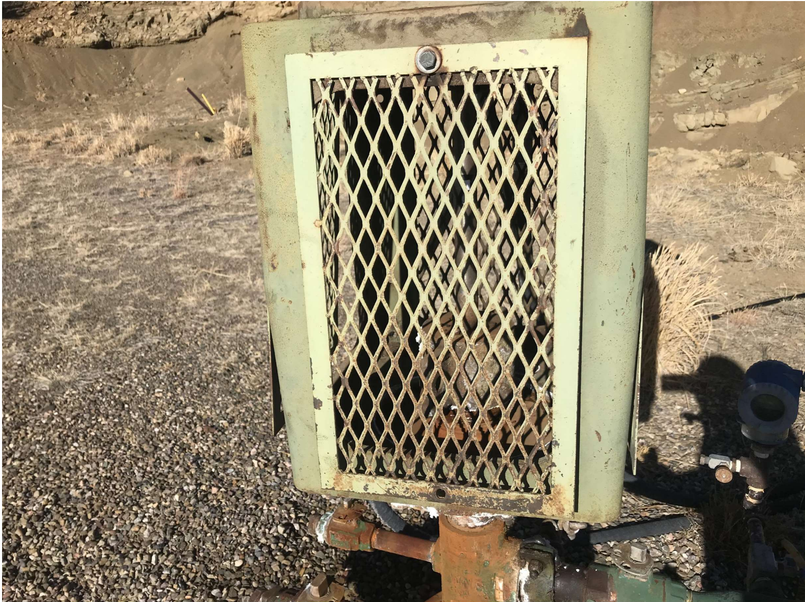
PHOTO 2: THE PACKINGS ON THE WELL HEAD WERE REPLACED TO ELIMINATE THE WATER LEAK.
