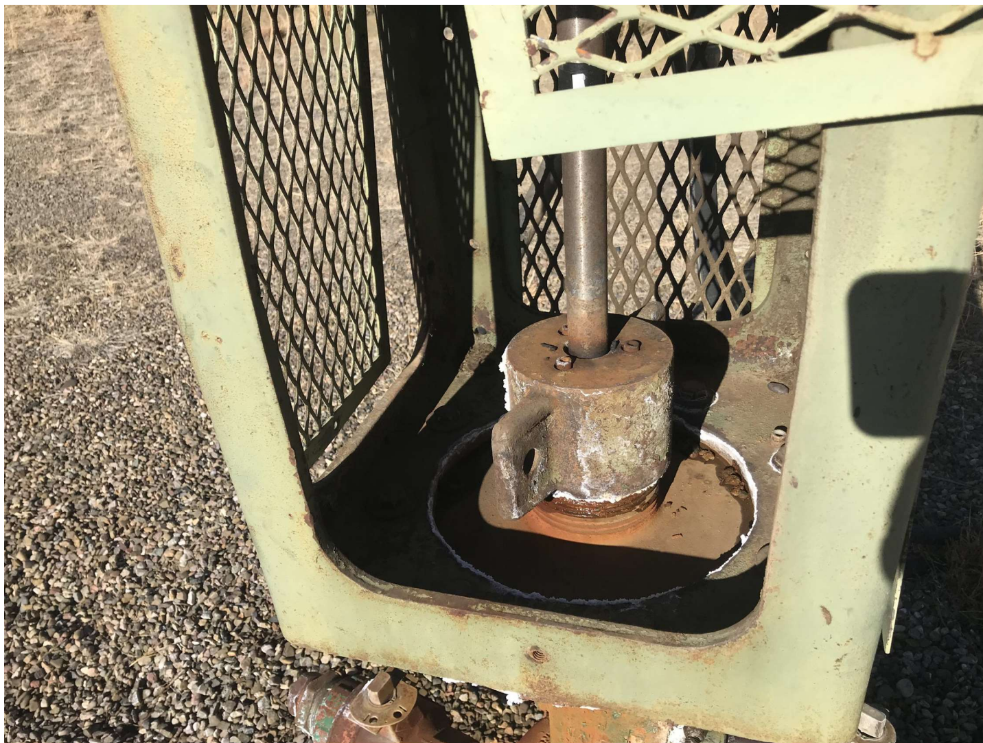
PHOTO 3: THE PACKINGS ON THE WELL HEAD WERE REPLACED TO ELIMINATE THE WATER LEAK.
