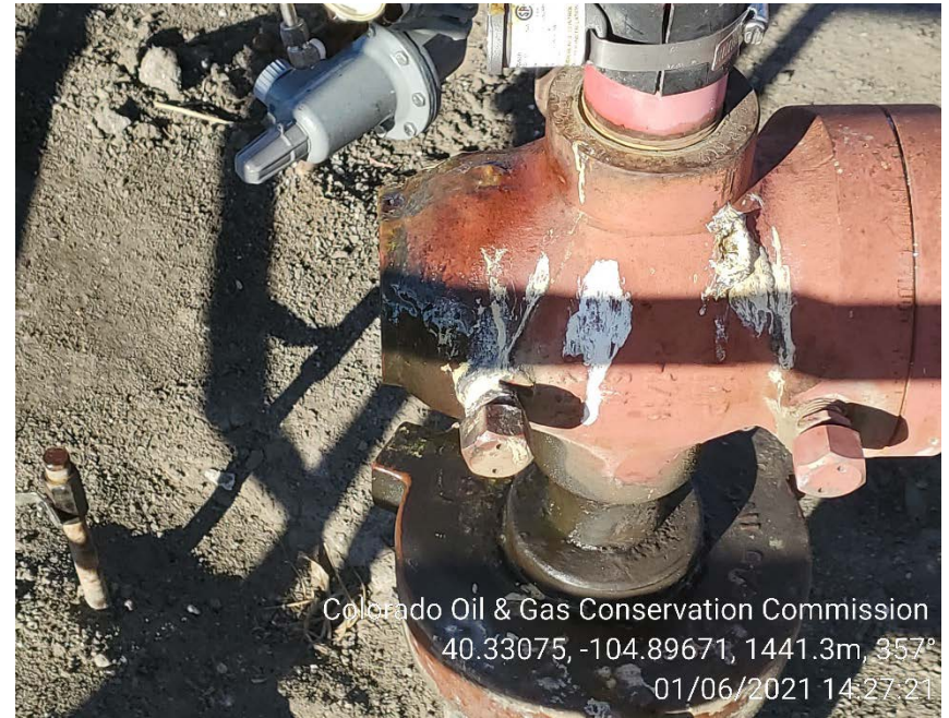
Lubricator leak
