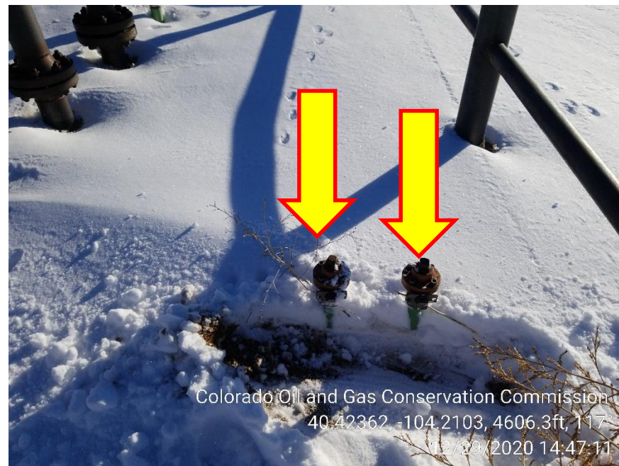
Photo 12 – Unmarked Riser
