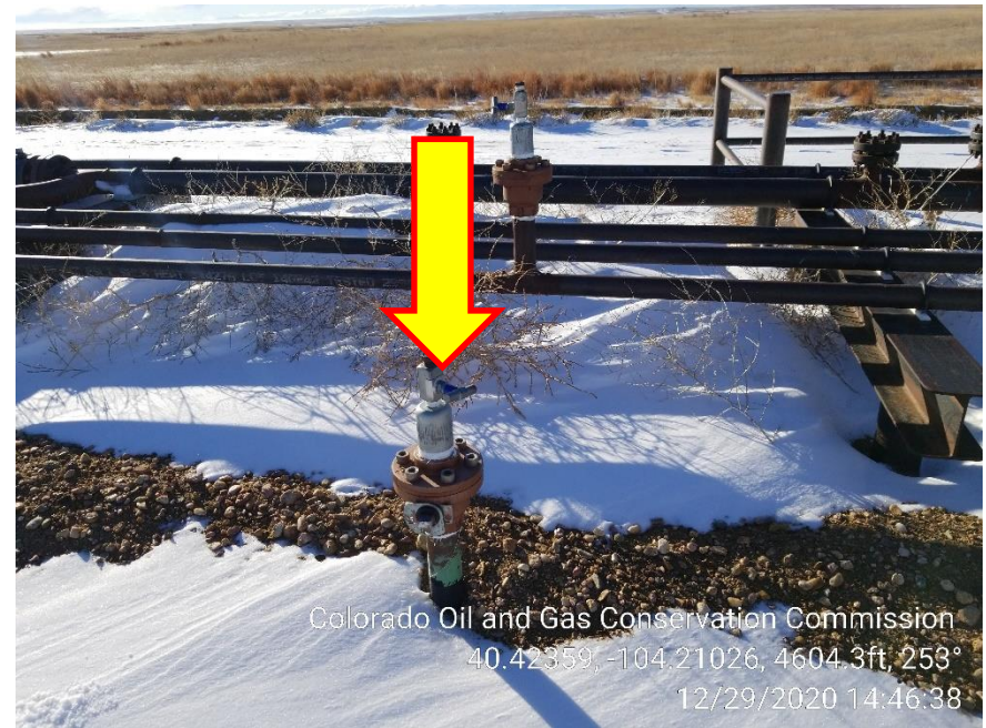
Photo 10 – Unmarked Riser
