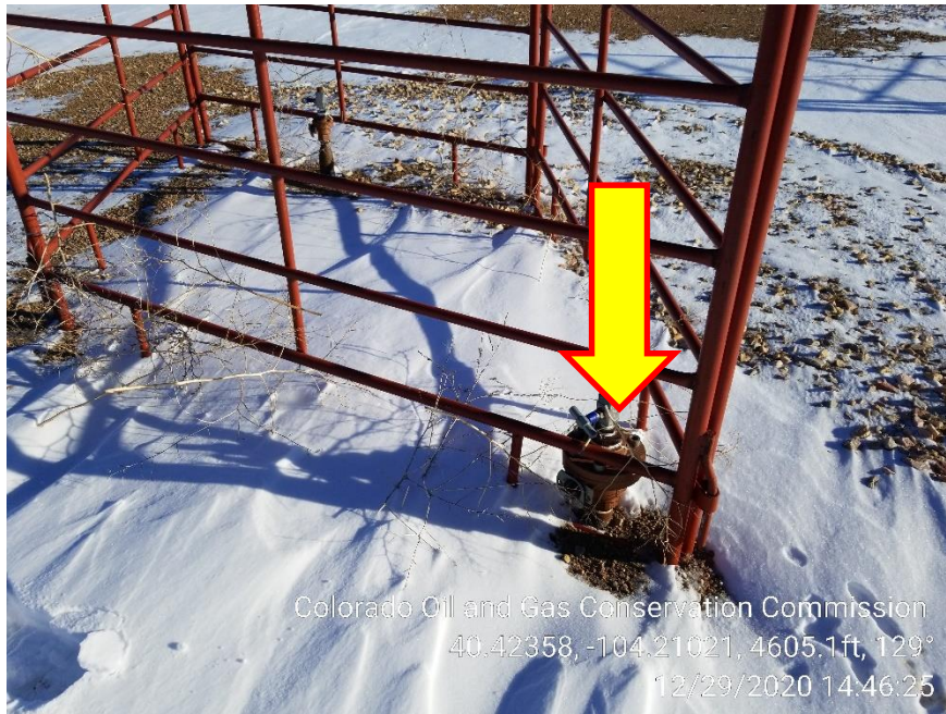
Photo 9 – Unmarked Riser
