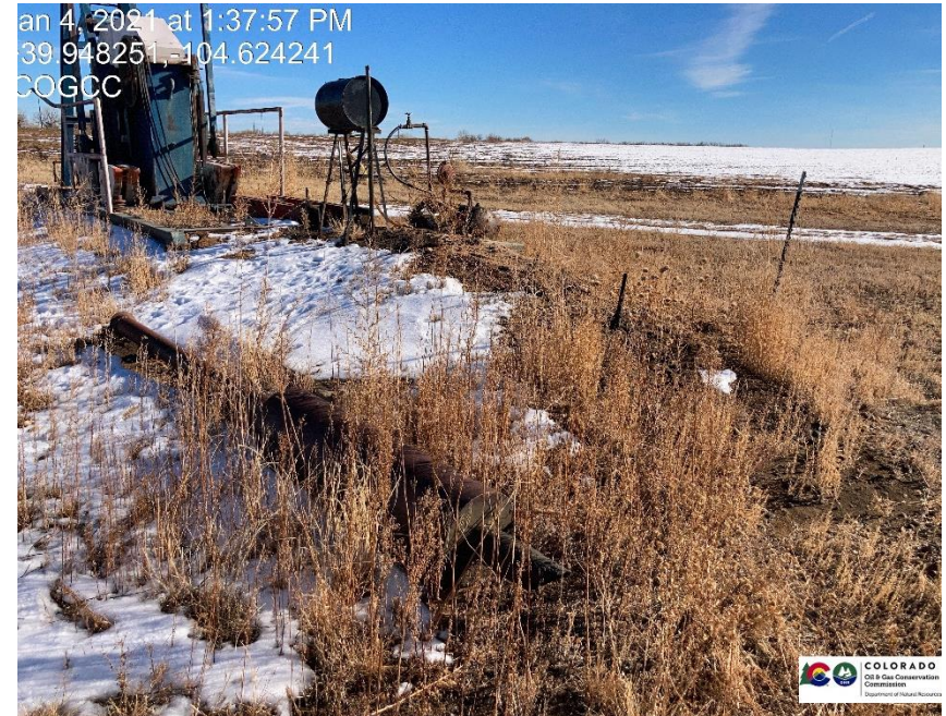
Pic 4 stained soil / weeds / no BMP under chemical tank
