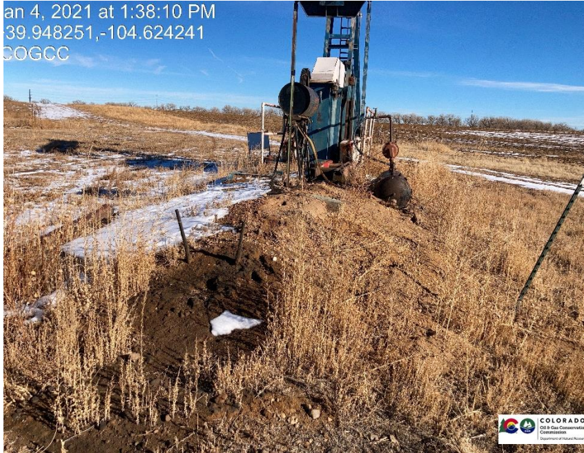
Pic 5 stained soil / no BMP under chemical tank/ weeds
