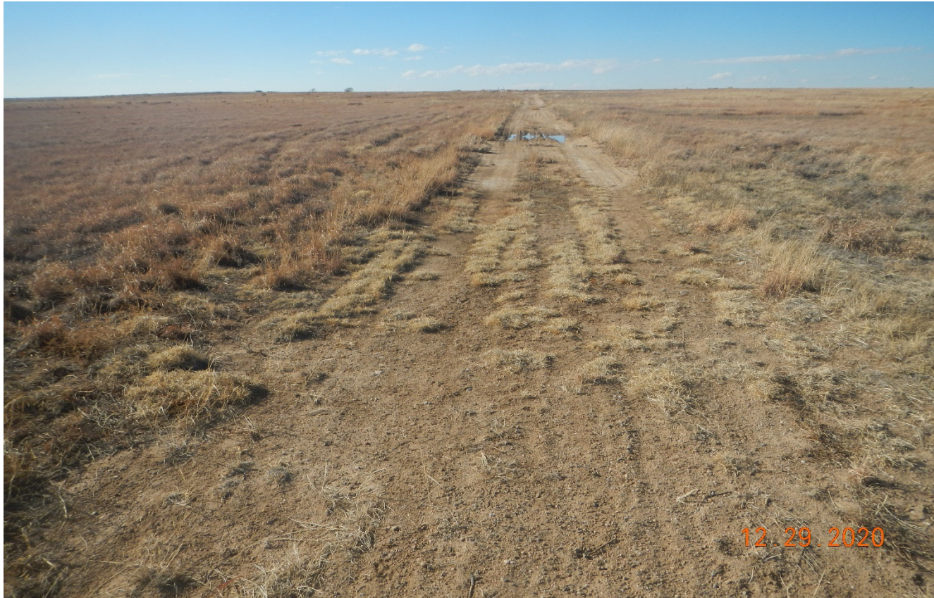
Photo 1. Facing west toward the access road. It appears the road may have been seeded however. It does not appear the road was decompacted by cross ripping to 18 inches.
