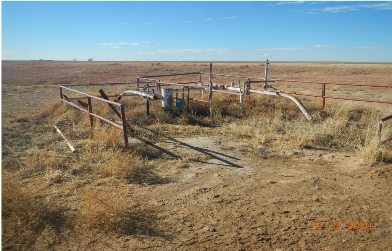
Photo 3. There is pipe risers and equipment that remain at the location. All equipment should have been removed within 3 months of abandonment.
