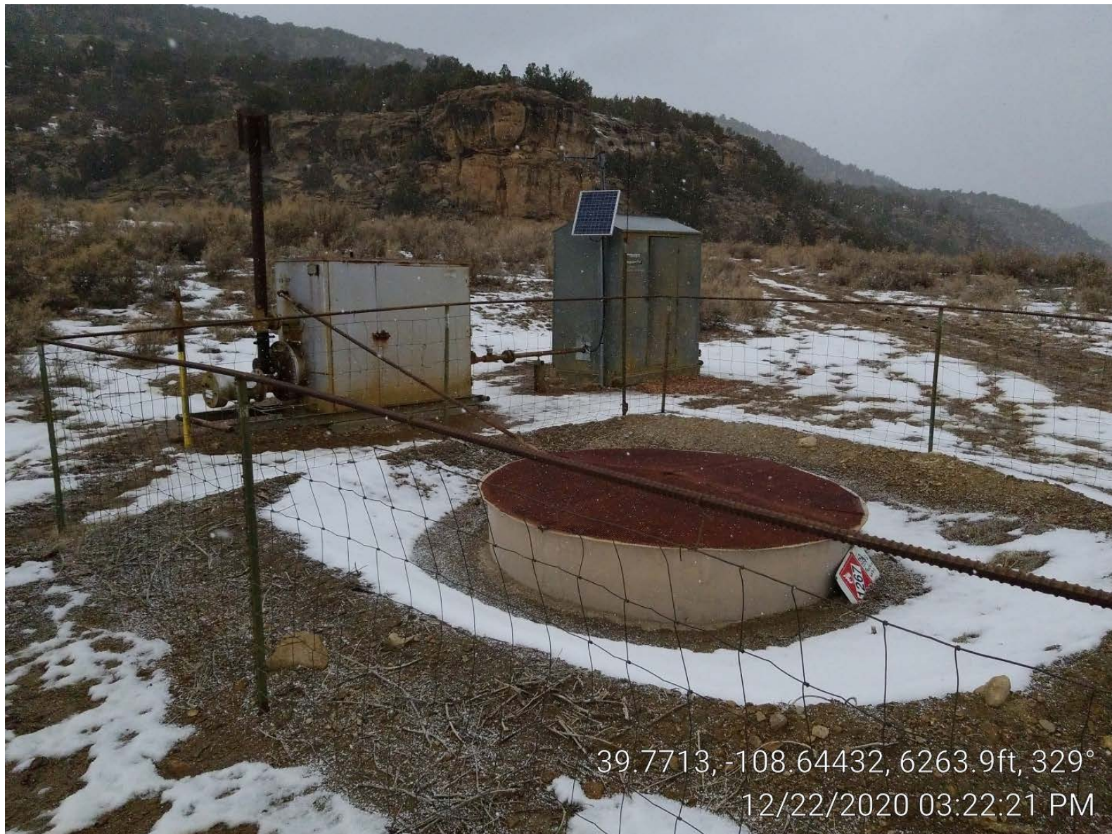
Photo 2. Tank, meter building, separator.
