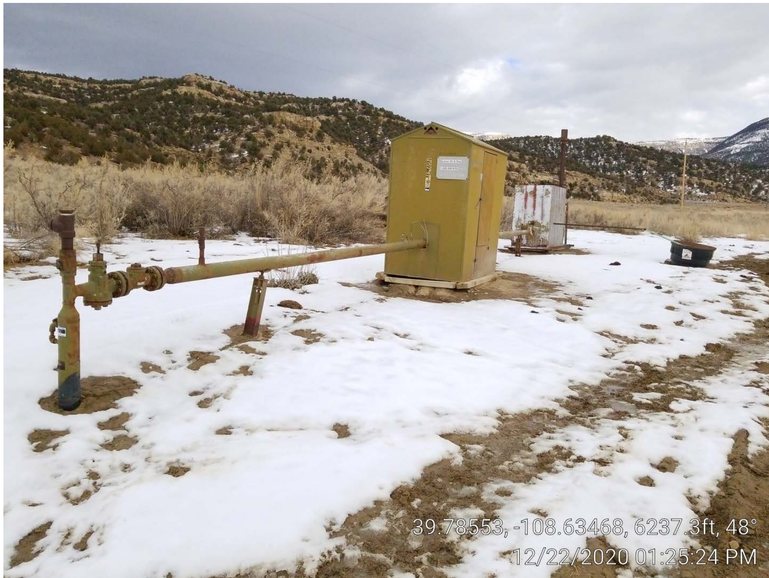
Photo 3. Meter building & separator.
