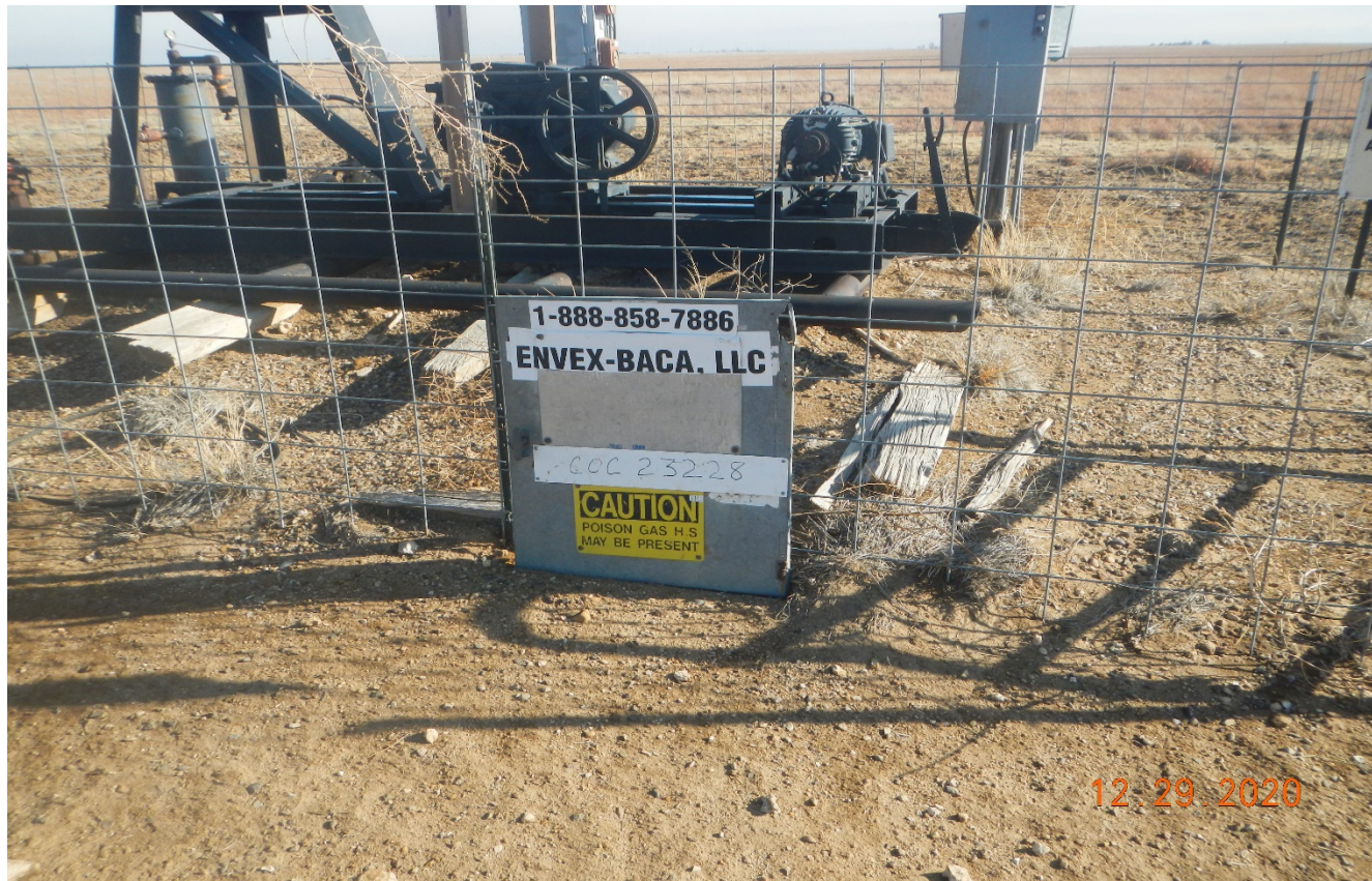
Photo 5. The well sign does not comply with 210.b.
