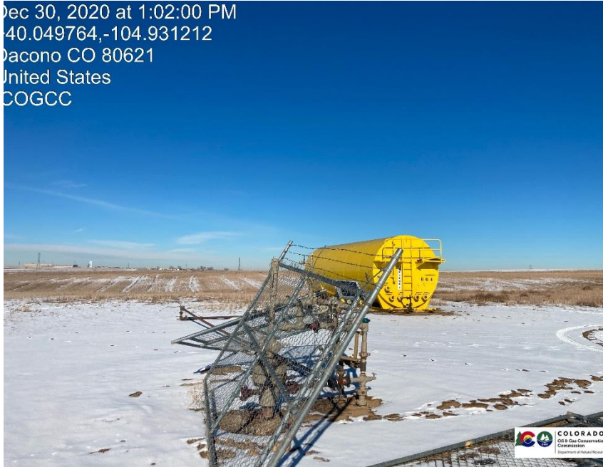
Pic 1 fence not installed correctly
