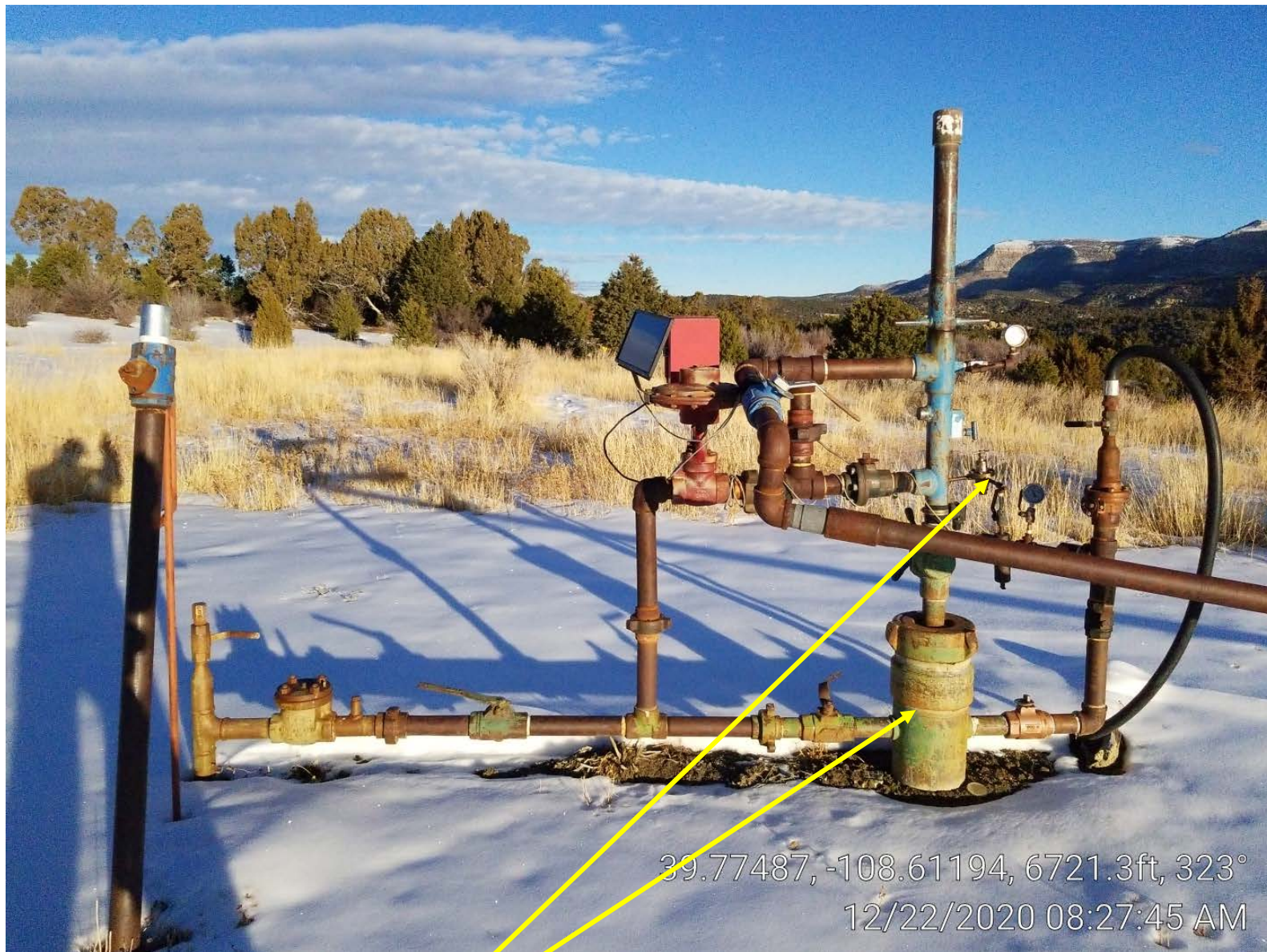
Photo 4. Well with gas leaks.
