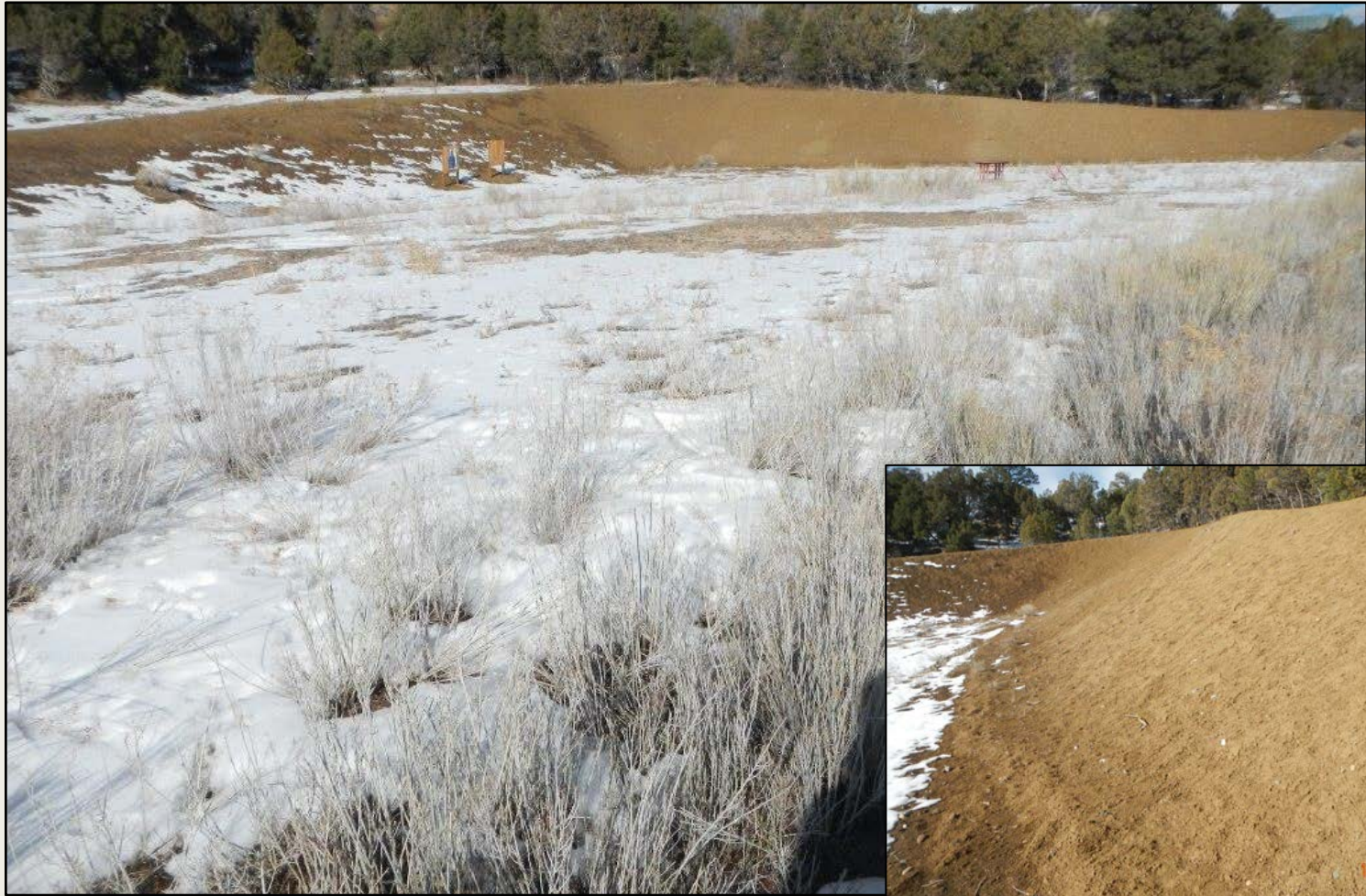
Photo 3. View of project area from the southeastern corner facing center. Inset shows a closeup of cut-slope. Little desirable vegetation. Per Condition of approval for variance, operator needs to establish vegetation and stabilize cut-slopes.
