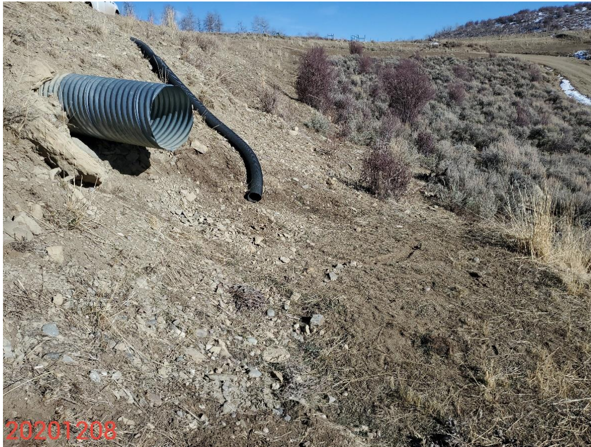
Photo 24: Photo taken from the access road north of the Location, facing north. Photo shows culvert and pipe. BMPs missing inlet/outlet protection and armoring in accordance with good engineering practices.
