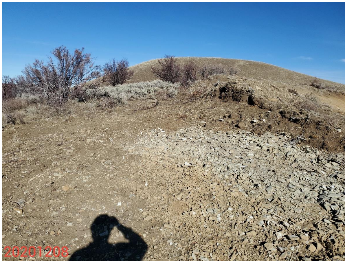
Photo 18: Photo taken from the northwest end of the Location, facing north. Photo erosion/head cutting evident on soil berms/stockpiles on the northwest end of the Location. BMPs remain missing or insufficient to protect/stabilize slopes/soils
