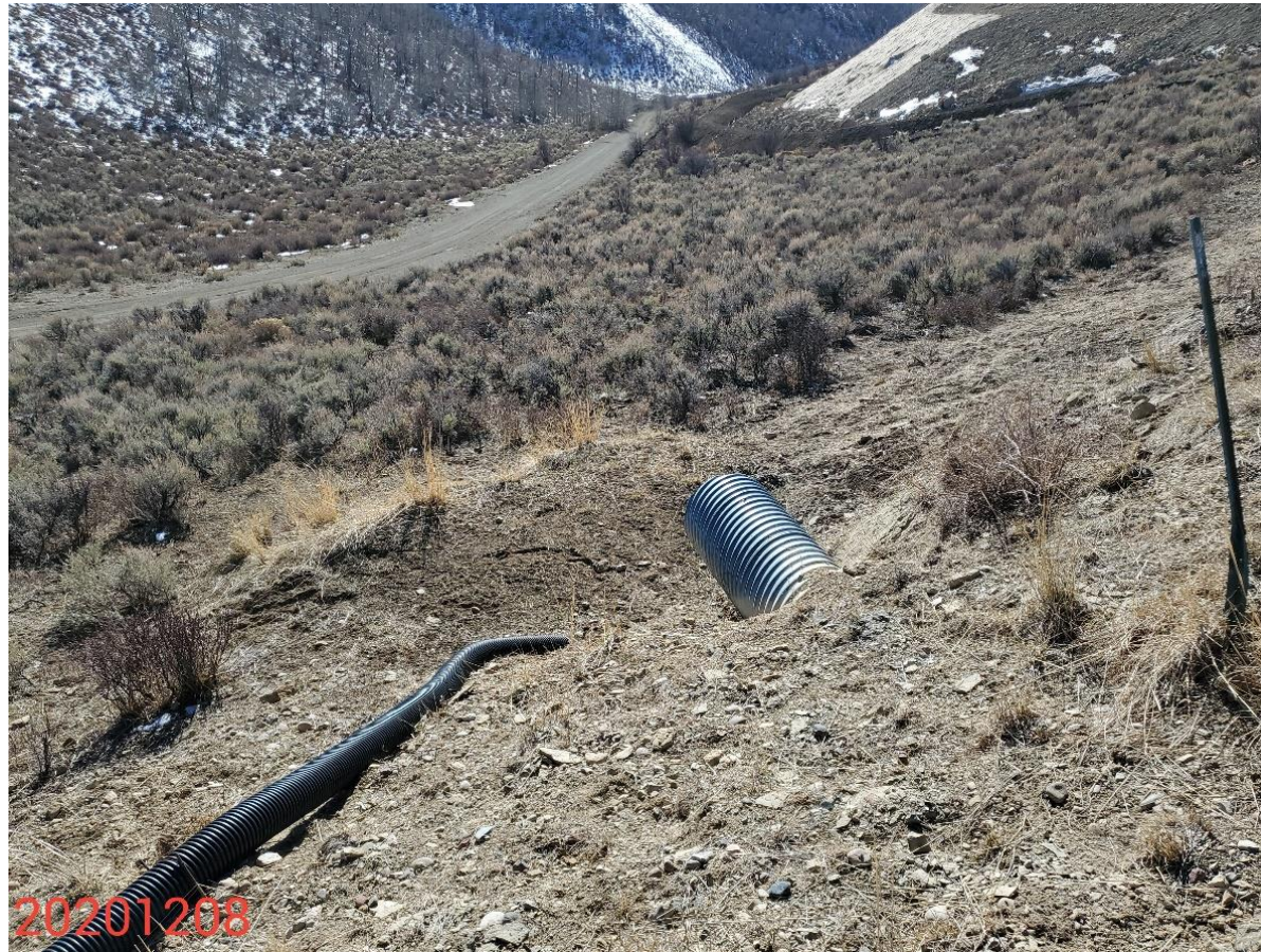
Photo 23: Photo taken from the access road north of the Location, facing southeast. Photo shows culvert and pipe. BMPs missing inlet/outlet protection and armoring in accordance with good engineering practices.
