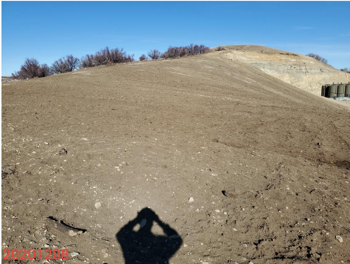
Photo 11: Photo taken from the southwest end of the Location, facing north. Photos 11-13 provide an overview of the Location from north, northeast to east. Photos show BMPs remain missing or insufficient to protect/stabilize slopes of the Location.
