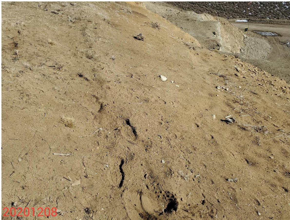
Photo 22: Photo taken from the northwest end of the Location, facing northeast. Photo shows BMPs remain missing or insufficient to protect/stabilize slopes/soils.
