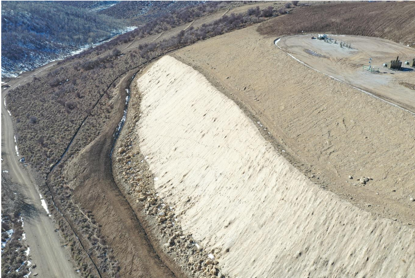
Photo 2: Photo taken with use of a sUAS. Photo taken from the east of the Location, facing south. Photo shows Operator installed erosion blankets on only a portion of the fill slopes. BMPs remain missing or insufficient to protect/stabilize slopes of the Location.
