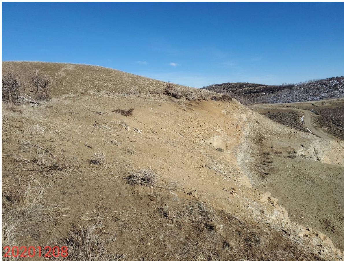
Photo 19: Photo taken from the northwest end of the Location, facing northeast. Photo shows BMPs remain missing or insufficient to protect/stabilize slopes/soils
