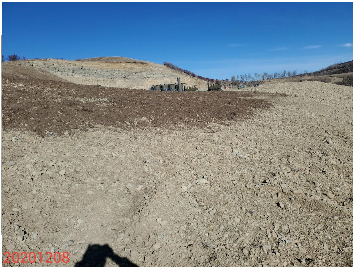
Photo 10: Photo taken from the southern areas of the Location, facing north. Photo shows BMPs remain missing or insufficient to protect/stabilize slopes of the Location.
