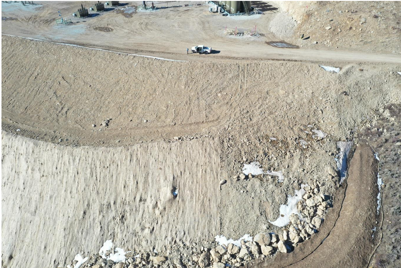
Photo 1: Photo taken with use of a sUAS. Photo taken from the east of the Location, facing west. Photo shows Operator installed erosion blankets on only a portion of the fill slopes. BMPs remain missing or insufficient to protect/stabilize slopes of the Location.
