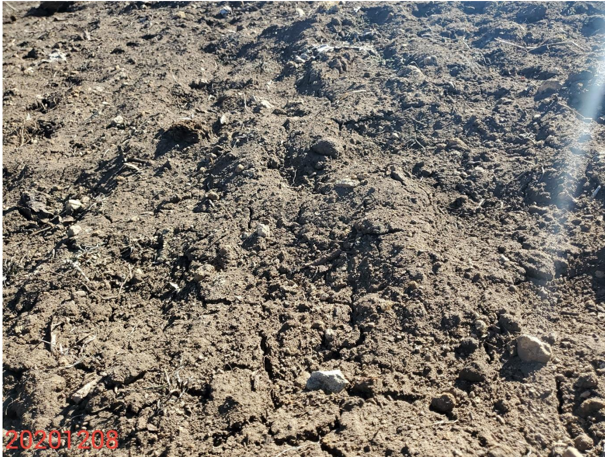
Photo 14: Photo taken from interim areas on the south end of the Location. Photo shows soil surface. Though interim reclamation activities including recontouring and regrading have been conducted, revegetation/seeding activities have not been conducted in accordance with Rule 1003.e.(2).
