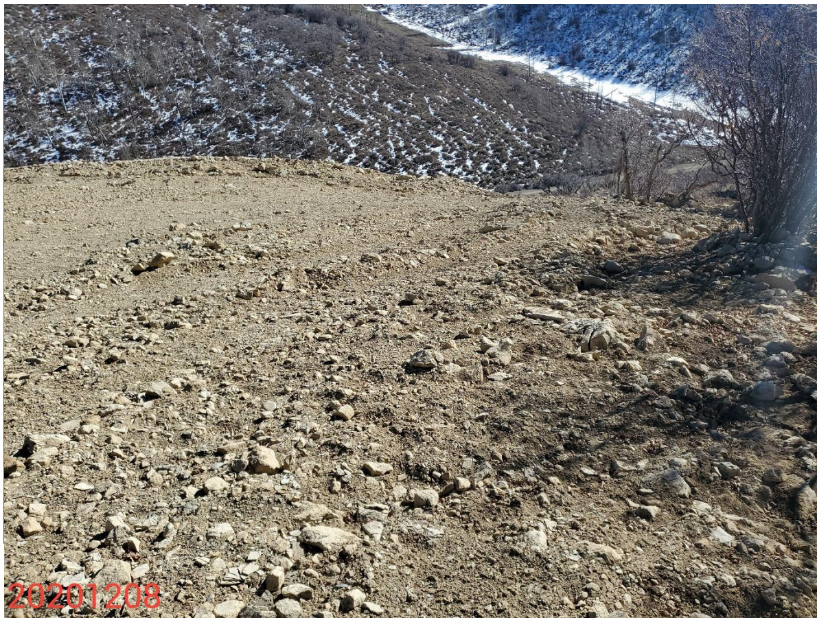
Photo 9: Photo taken from the southeastern areas of the Location, facing east. Photo shows BMPs remain missing or insufficient to protect/stabilize slopes of the Location.
