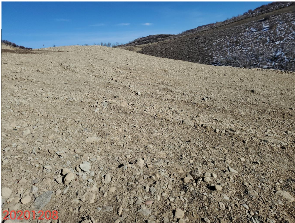
Photo 8: Photo taken from the southeastern areas of the Location, facing north. Photo shows BMPs remain missing or insufficient to protect/stabilize slopes of the Location.
