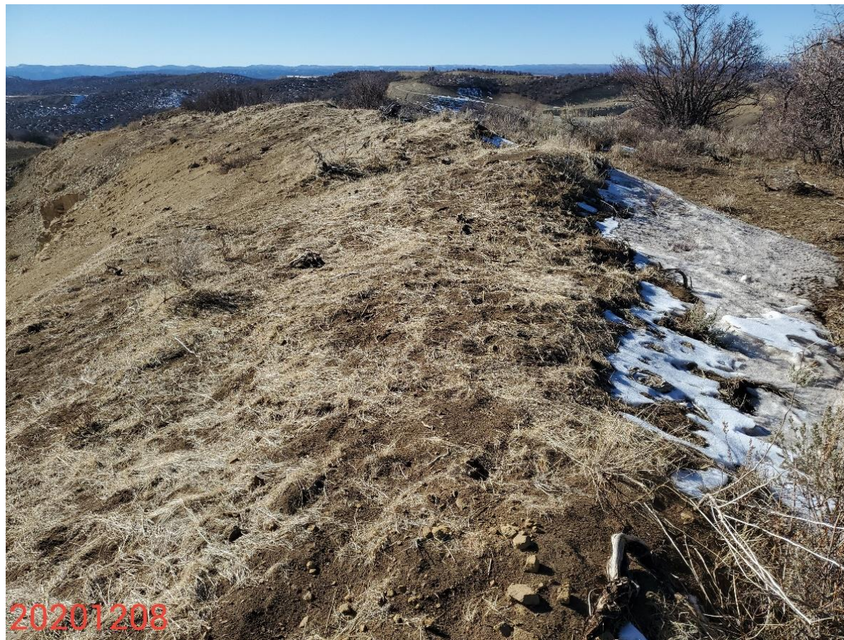
Photo 21: Photo taken from the northwest end of the Location, facing south. Photo erosion/head cutting evident on soil berms/stockpiles on the northwest end of the Location. BMPs remain missing or insufficient to protect/stabilize slopes/soils.
