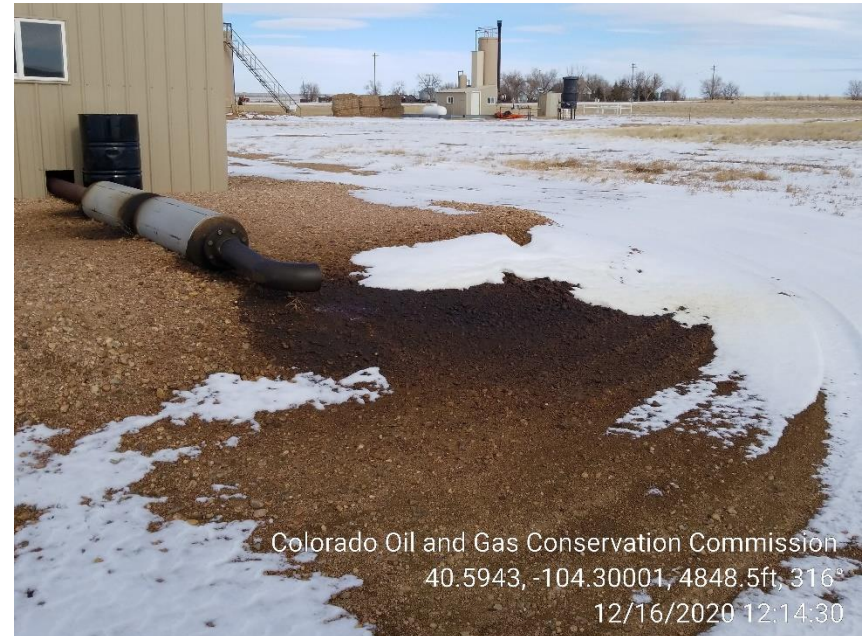
Photo 4 – Stained Soil at Engine Exhaust
