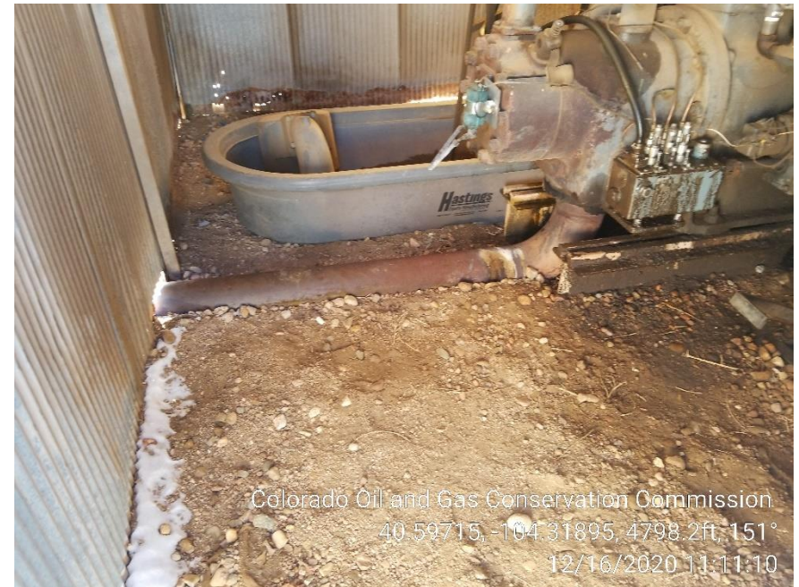
Photo 8 – Stained Soil at Gas Engine
