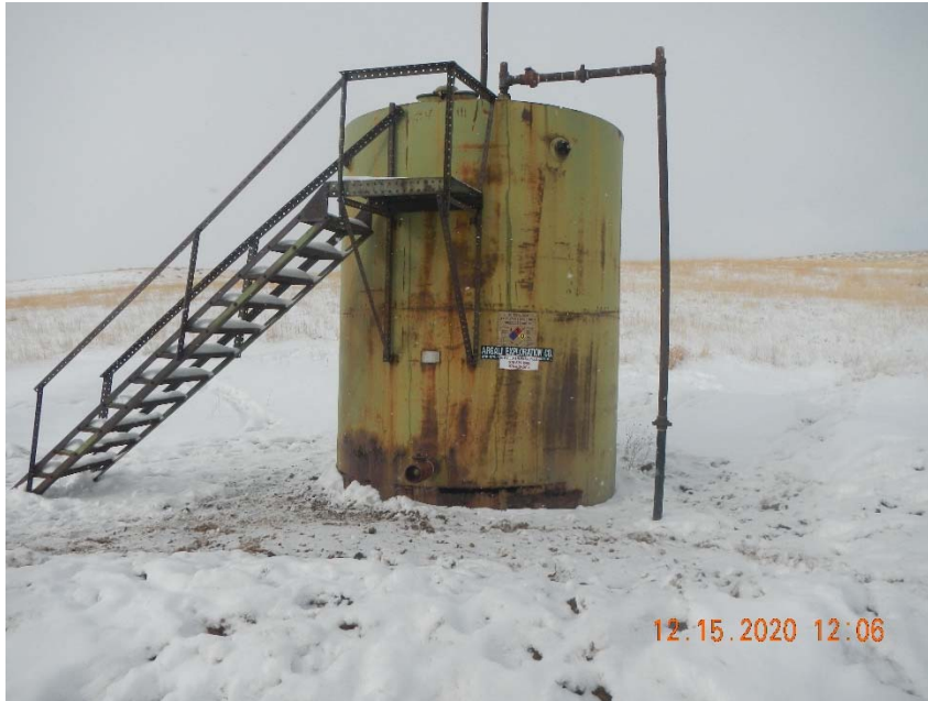
Photo 3. Produced water tank with corrosion holes along bottom side.
