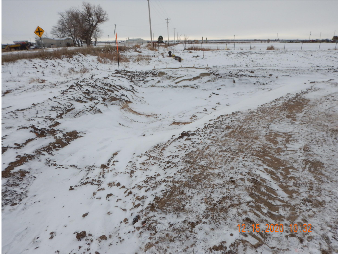
Photo 7. Photo taken from the southeastern location, facing South. Photo illustrates the sediment trap installed with a temporarily stabilized outlet. This will likely be sufficient for winter conditions but this will not be sufficient for the monsoon season and to protect the irrigation ditch 14' feet to east of the location.
