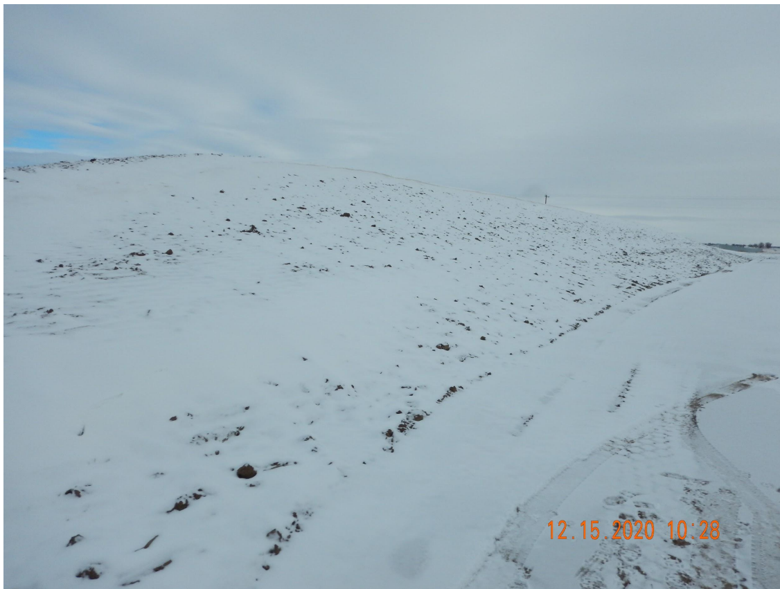
Photo 5. Photo taken from the northwestern location, facing Northeast. Photo illustrates the Operator has temporarily stabilized the topsoil with equipment tracking.
