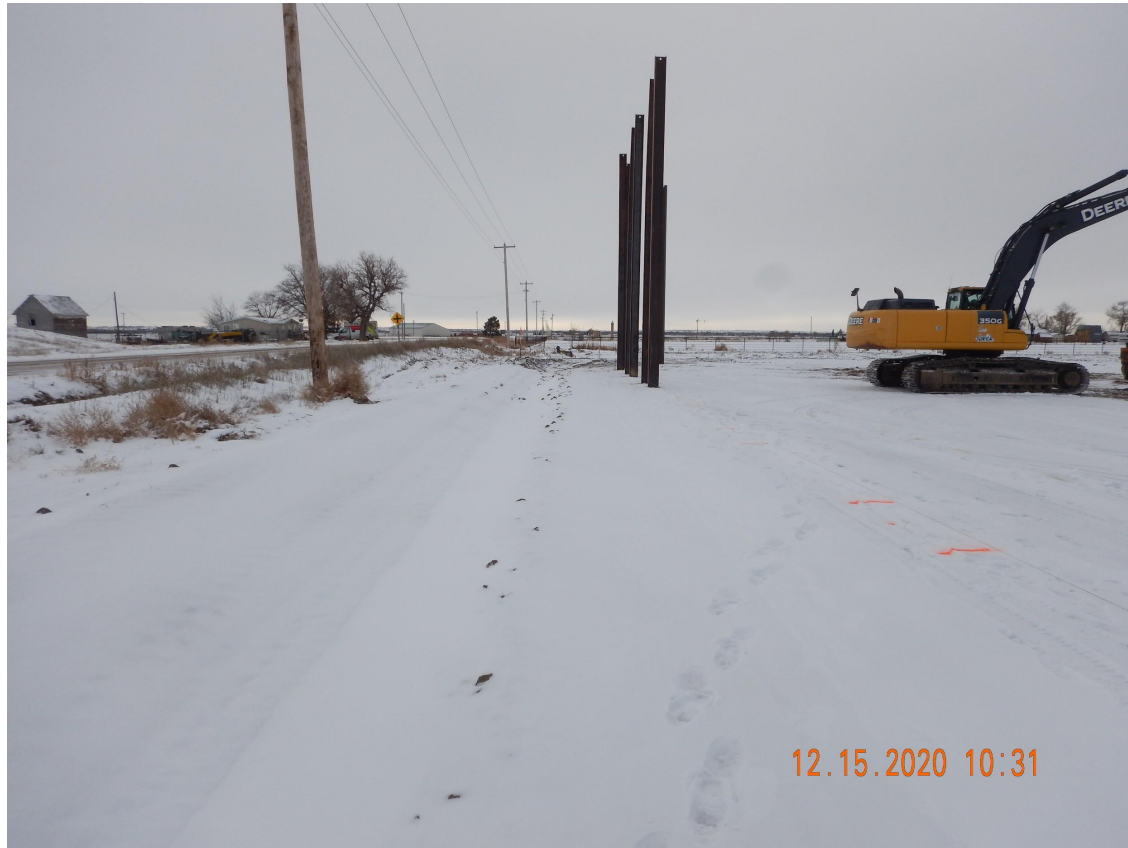
Photo 1. Photo taken from the entrance of location, facing South. Photo illustrates has installed a ditch and berm BMP around the entire perimeter of location in conjunction with a sediment trap. Sound wall installation was being conducted at the time of this inspection. At the time of this inspection, there was no observed Form 2A posted at location.
