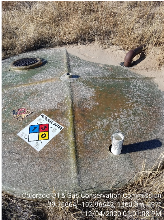
11. Overflowing to 98% buried tank
