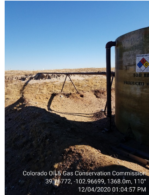
8. Water tank with overflow to pit
