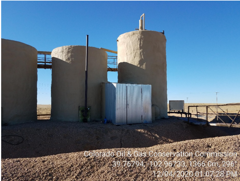
5. Gun barrel and pump shed
