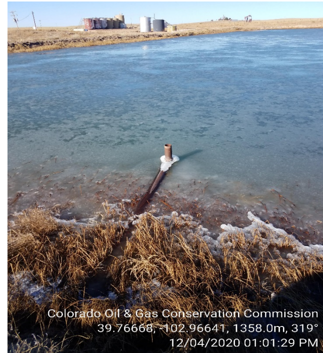
10. Overflow from pit to buried tank
