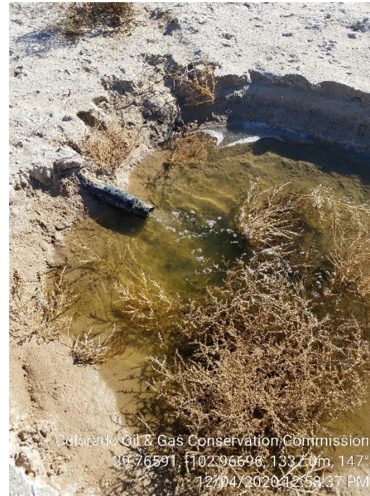
12. Overflow from buried tank to surface discharge.
