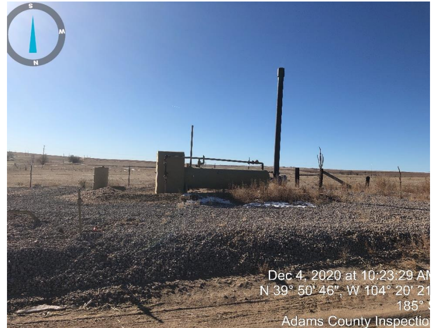
Photo #2 Separator and unmarked risers.
