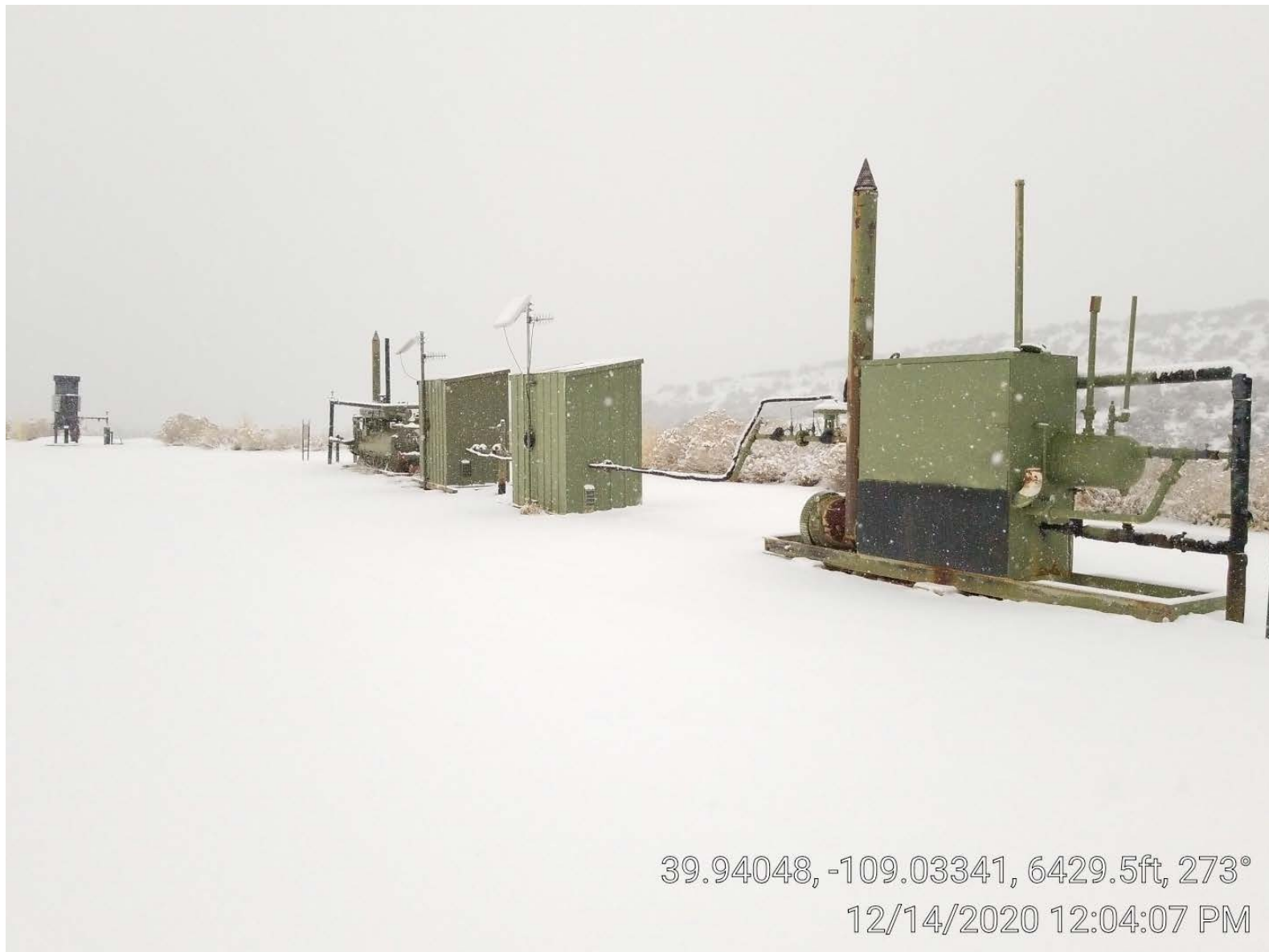
Photo 5. Separators, meter buildings, combustor.
