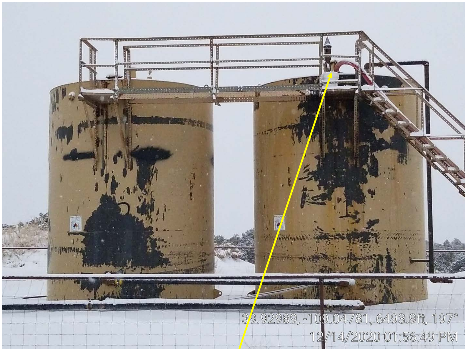
Photo 4. Water tanks. Open hatch gas venting.
