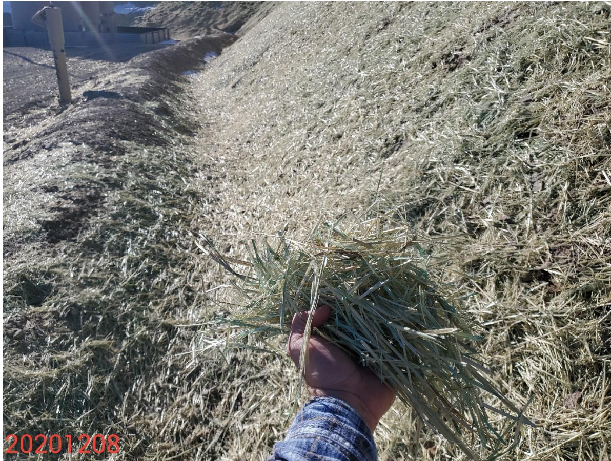
Photo 3: Photo taken from the north end of the Location, facing west. Operator applied mulch to the slopes; BMP insufficient to stabilize/protect slopes and/or has not been installed on slope in accordance with good engineering practices.
