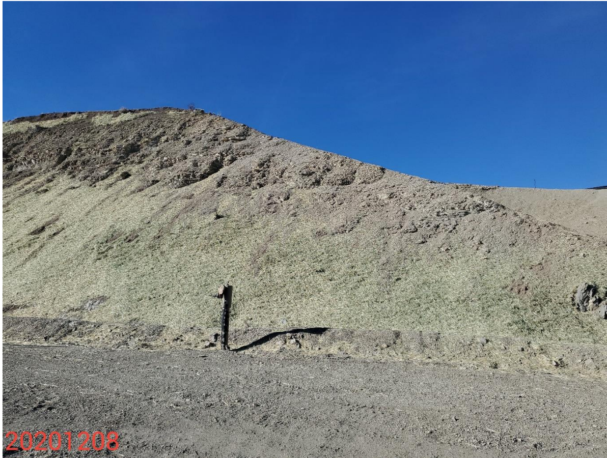
Photo 2: Photo taken from the north end of the Location, facing northwest. Operator applied mulch to the slopes; BMP insufficient to stabilize/protect slopes and/or has not been installed on slope in accordance with good engineering practices.
