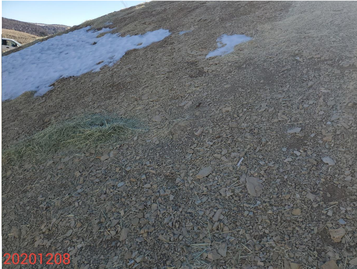
Photo 7: Photo taken from the north end of the Location, facing west. Operator applied mulch to the slopes; BMP insufficient to stabilize/protect slopes and/or has not been installed on slope in accordance with good engineering practices.
