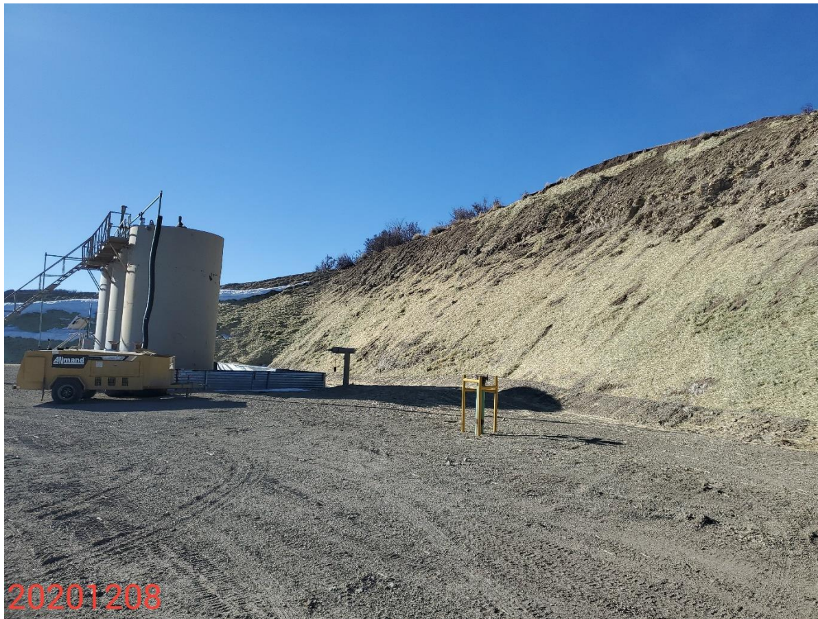
Photo 1: Photo taken from the north end of the Location, facing northwest. Operator applied mulch to the slopes; BMP insufficient to stabilize/protect slopes and/or has not been installed on slope in accordance with good engineering practices.
