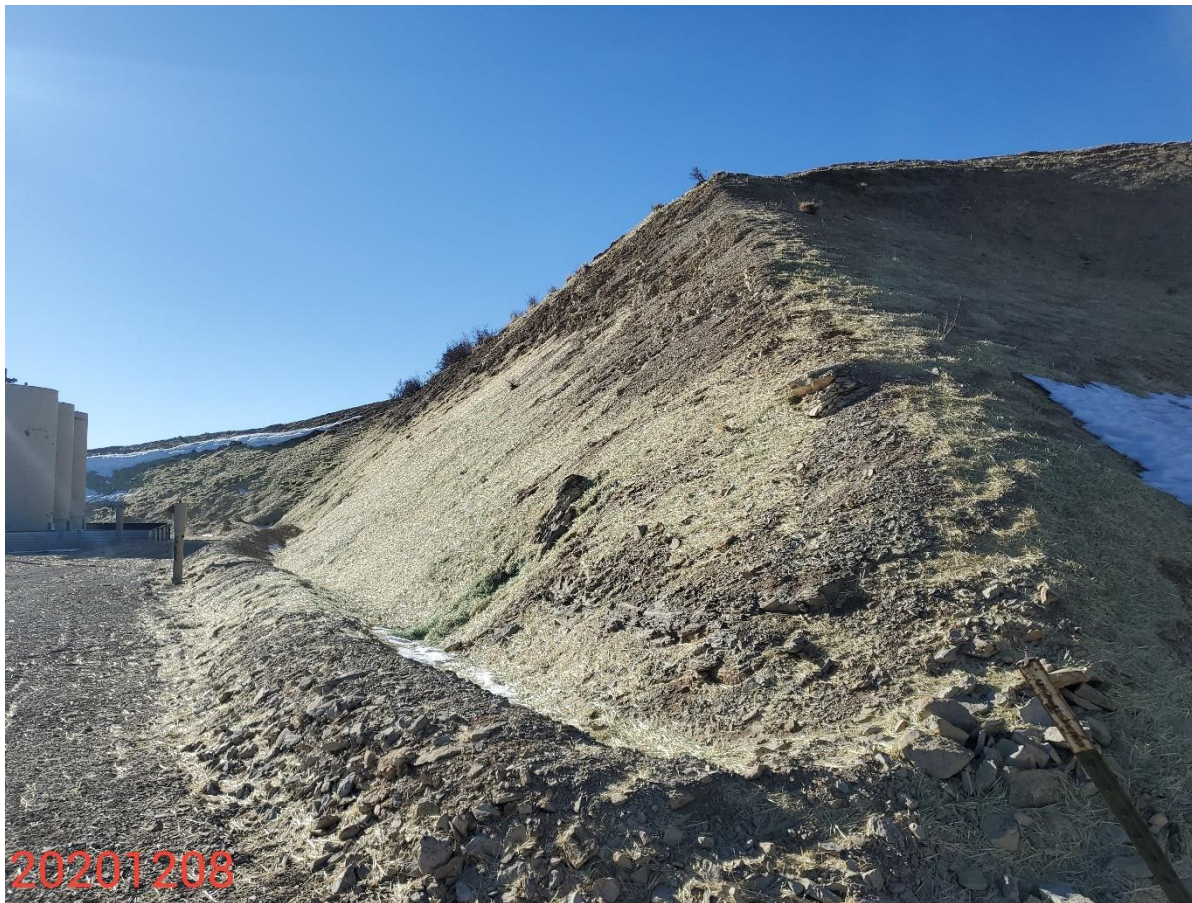
Photo 4: Photo taken from the north end of the Location, facing west. Operator applied mulch to the slopes; BMP insufficient to stabilize/protect slopes and/or has not been installed on slope in accordance with good engineering practices.
