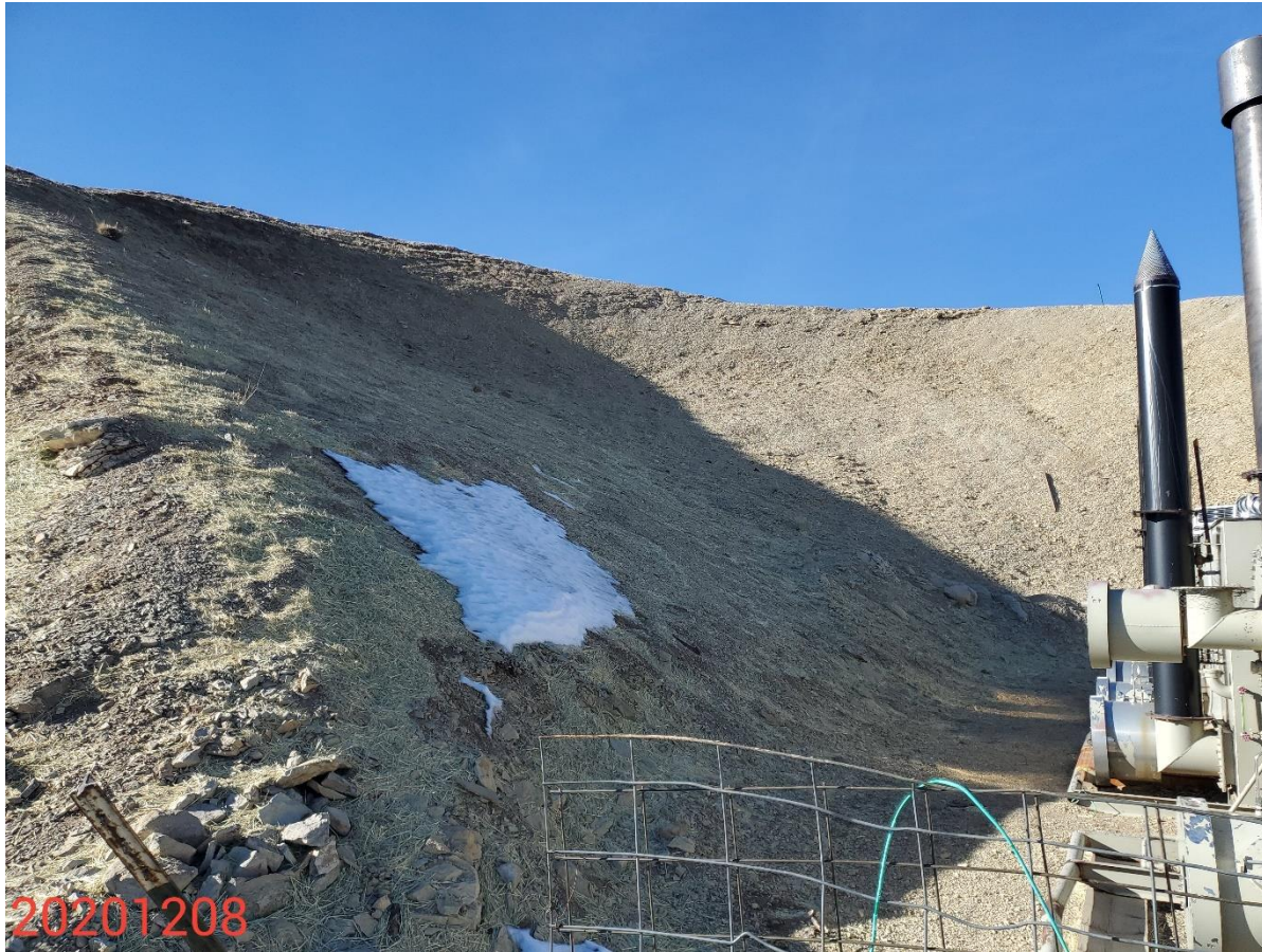
Photo 5: Photo taken from the north end of the Location, facing north. Photo shows areas of cut slope on the north end of the Location where BMPs have not been implemented to stabilize or protect cutslopes. .
