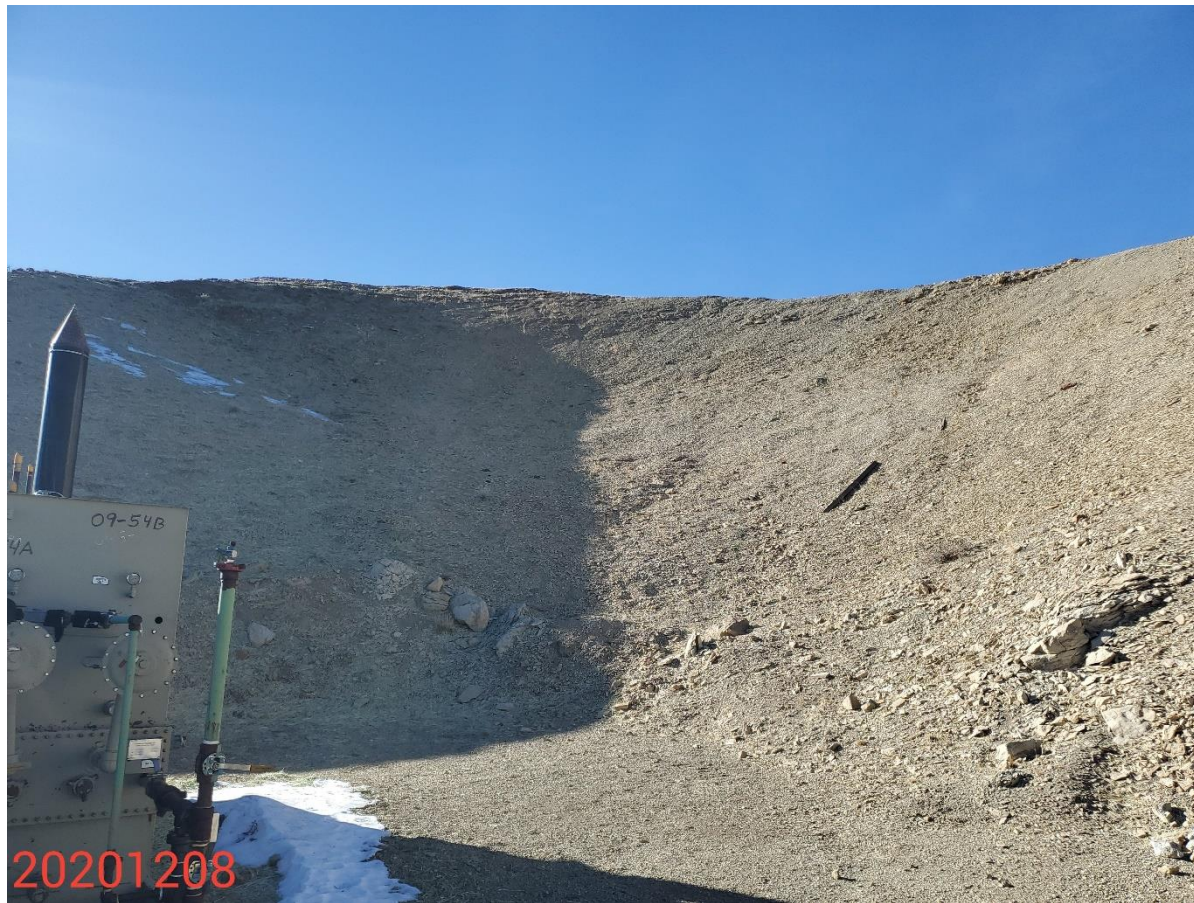
Photo 6: Photo taken from the north end of the Location, facing north. Photo shows areas of cut slope on the north end of the Location where BMPs have not been implemented to stabilize or protect cutslopes.
