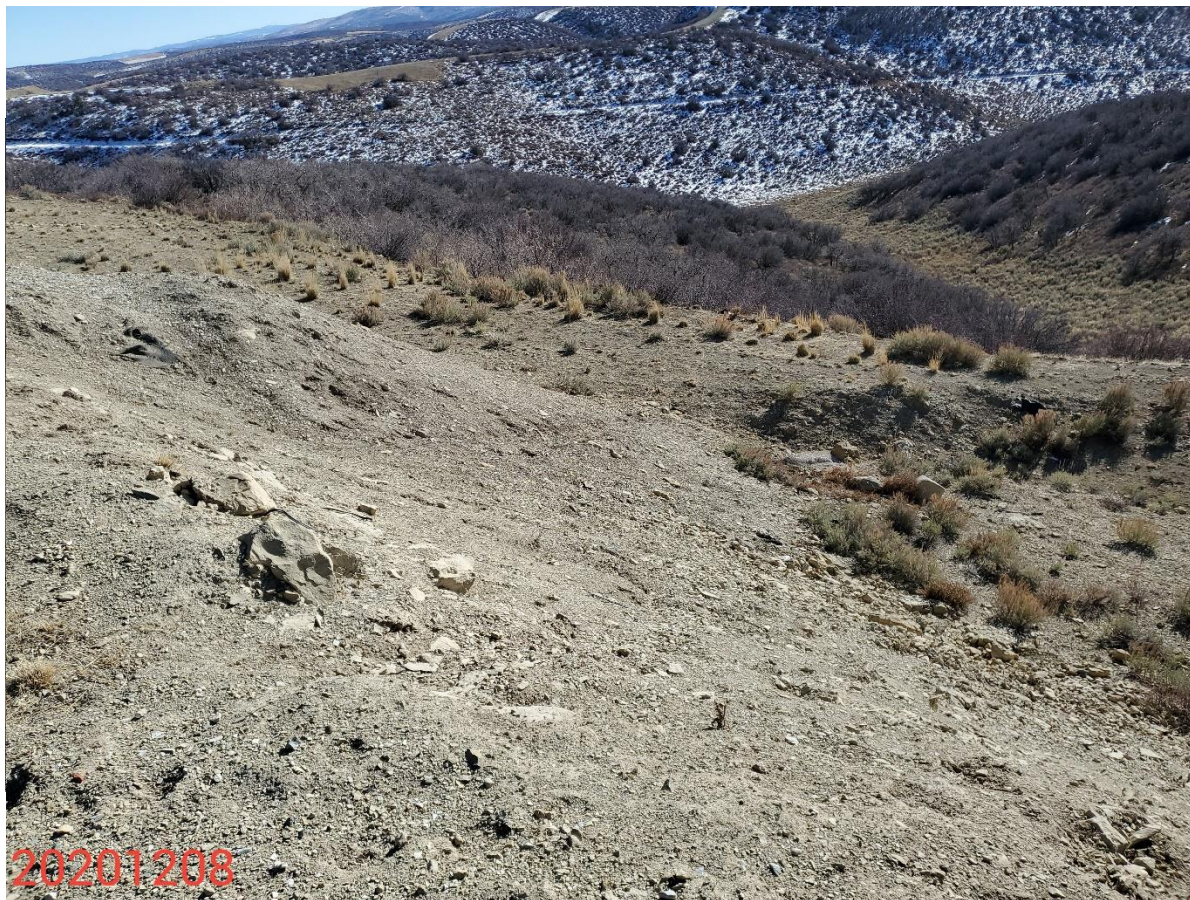
Photo 10: Photo taken from the southwest end of the Location, facing southeast. Photo shows BMPs to stabilize/protect slopes, and prevent off-site sediment transport are missing, or insufficient.
