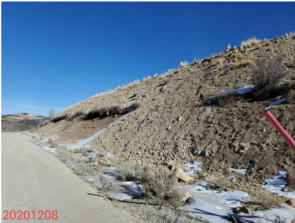
Photo 11: Photo taken from the access road on the north end of the Location, facing northwest. Photo shows BMPs to stabilize/protect slopes, and prevent off-site sediment transport are missing, or insufficient.
