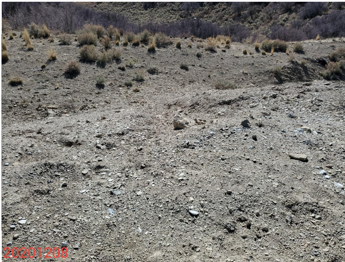
Photo 9: Photo taken from the southwest end of the Location, facing south. Photo shows BMPs to stabilize/protect slopes, and prevent off-site sediment transport are missing, or insufficient.
