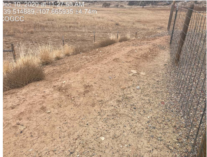
Lack of stabilization on slope next to separators
