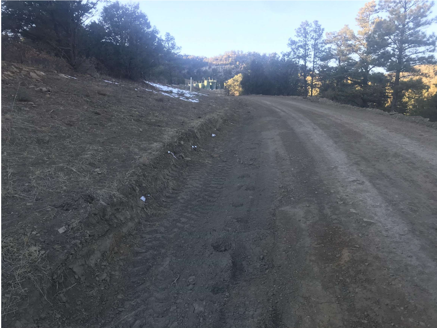
PHOTO 6: THE EROSION IN THE BAR DITCH WAS BACK FILLED AND COMPACTED WITH THE TIRE ON THE BACKHOE.
