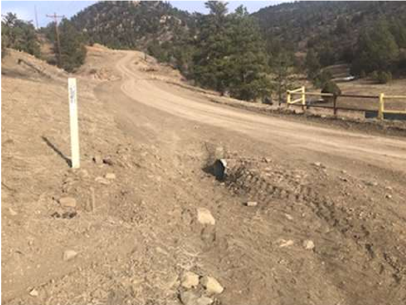
PHOTO 4: THE SEDIMENT ACCUMULATION WAS REMOVED FROM THE CULVERT INLET ALONG THE MAIN ROAD IN LOPEZ CANYON.
