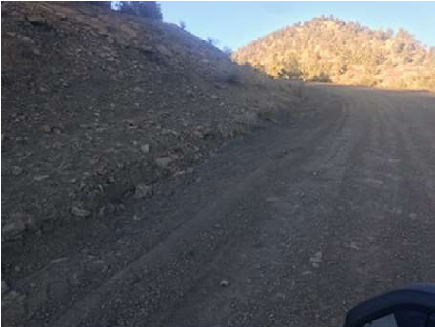
PHOTO 5: THE EROSION IN THE BAR DITCH WAS BACK FILLED AND COMPACTED WITH THE TIRE ON THE BACKHOE.
