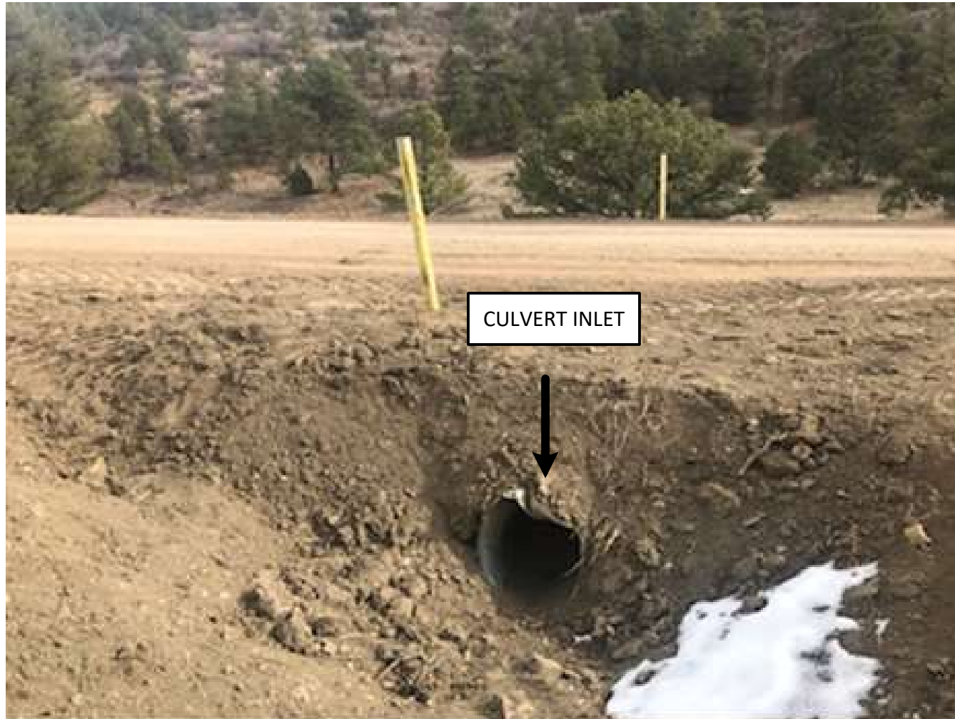
PHOTO 2: THE SEDIMENT ACCUMULATION WAS REMOVED FROM THE CULVERT INLET ALONG THE MAIN ROAD IN LOPEZ CANYON.
