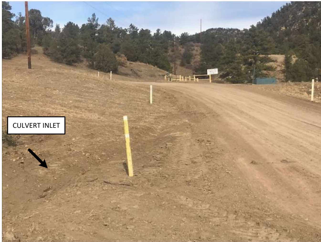
PHOTO 1: THE SEDIMENT ACCUMULATION WAS REMOVED FROM THE CULVERT INLET ALONG THE MAIN ROAD IN LOPEZ CANYON.
