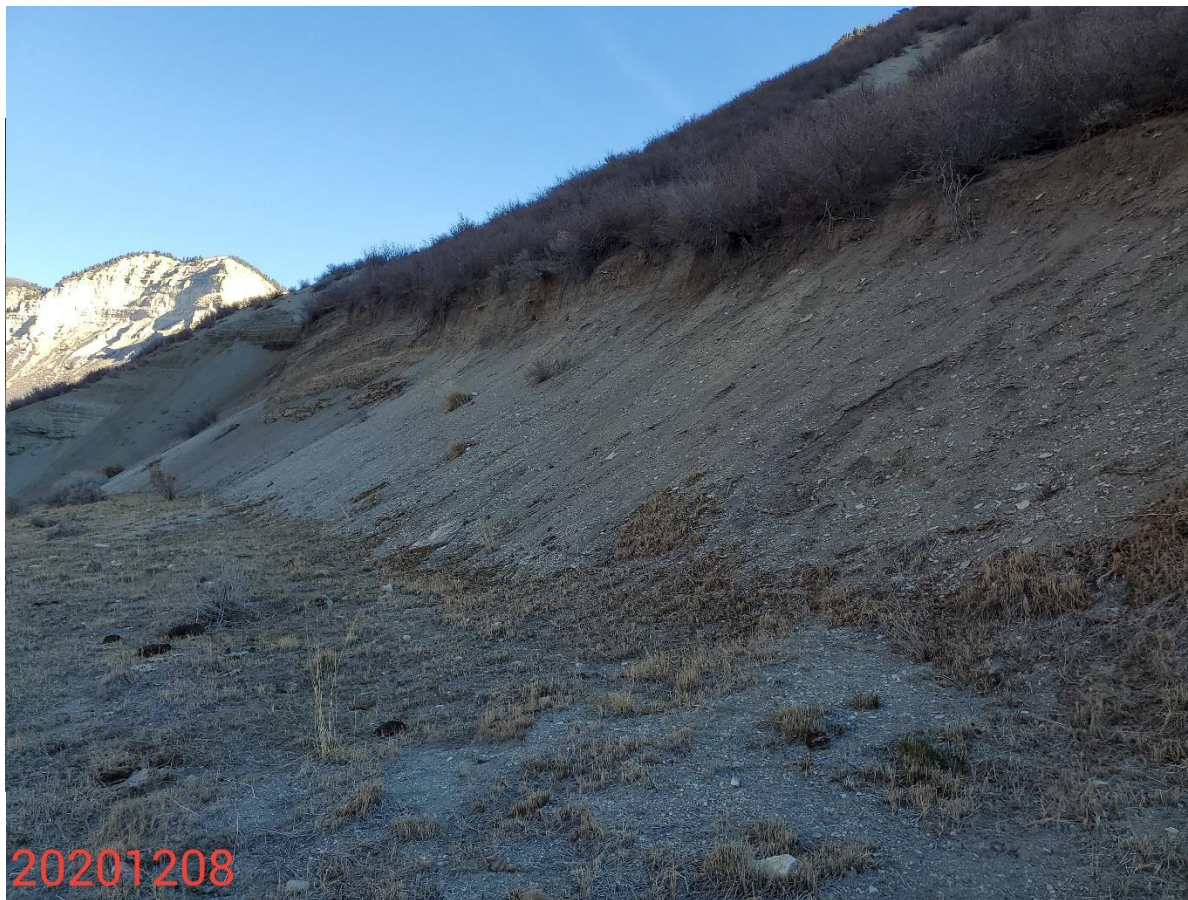
Photo 7: Photo taken from the southeast end of the Location, facing northeast. Photo shows BMPs to stabilize and protect cut slopes remain missing or insufficient.
