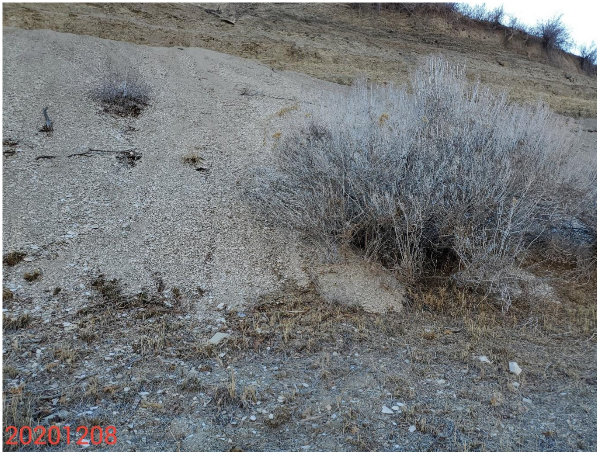
Photo 5: Photo taken from the east end of the Location, facing east. Photo shows BMPs to stabilize and protect cut slopes remain missing or insufficient.
