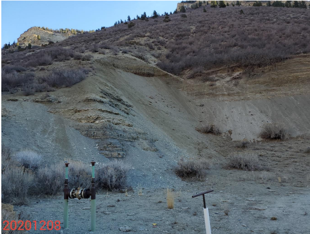
Photo 3: Photo taken from the north end of the Location, facing east. Photo shows BMPs to stabilize and protect cut slopes remain missing or insufficient. .
