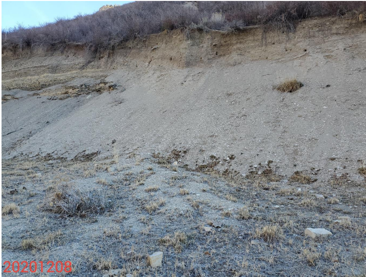
Photo 6: Photo taken from the east end of the Location, facing northeast. Photo shows BMPs to stabilize and protect cut slopes remain missing or insufficient.
