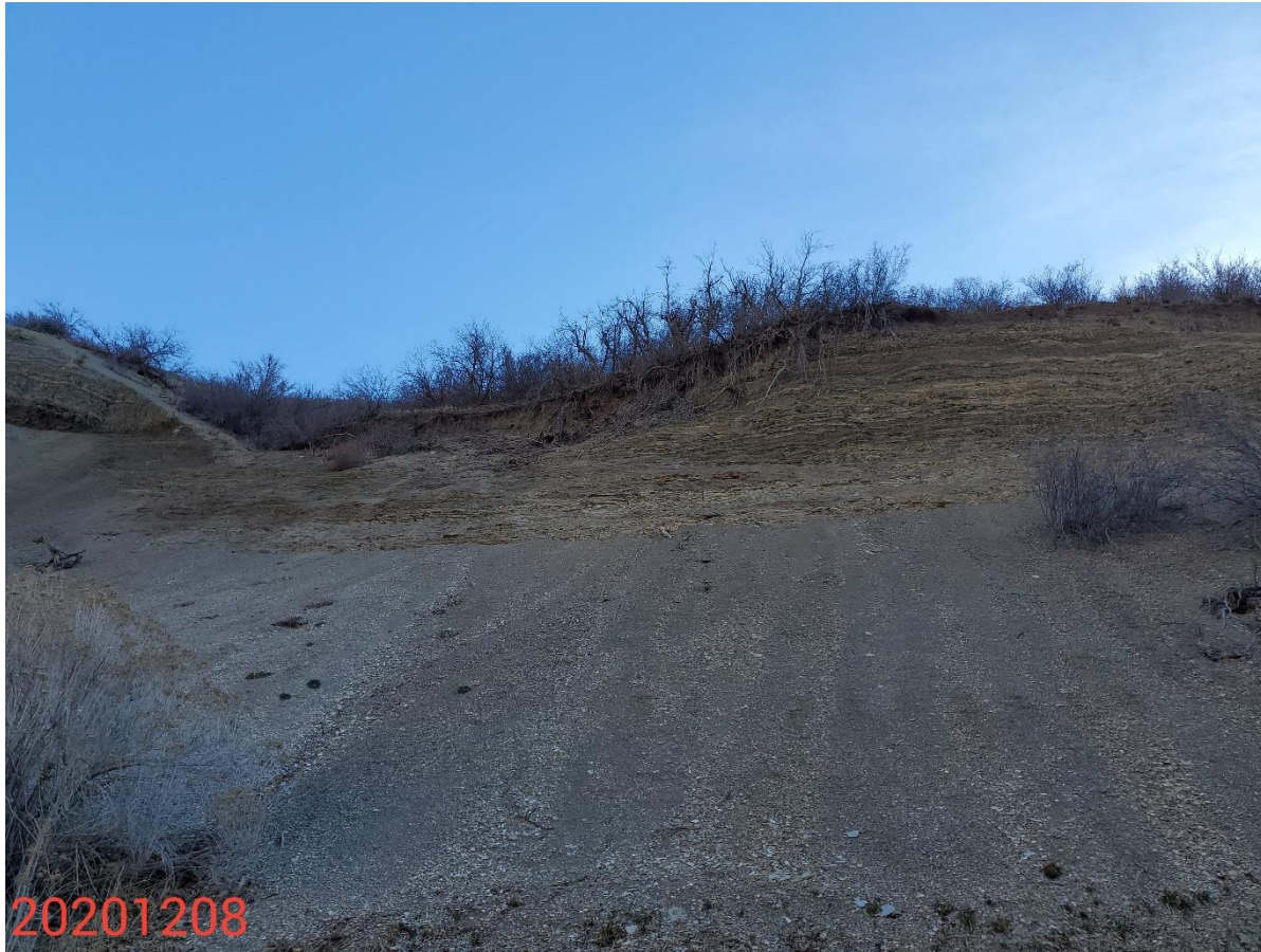
Photo 4: Photo taken from the east end of the Location, facing east. Photo shows BMPs to stabilize and protect cut slopes remain missing or insufficient.
