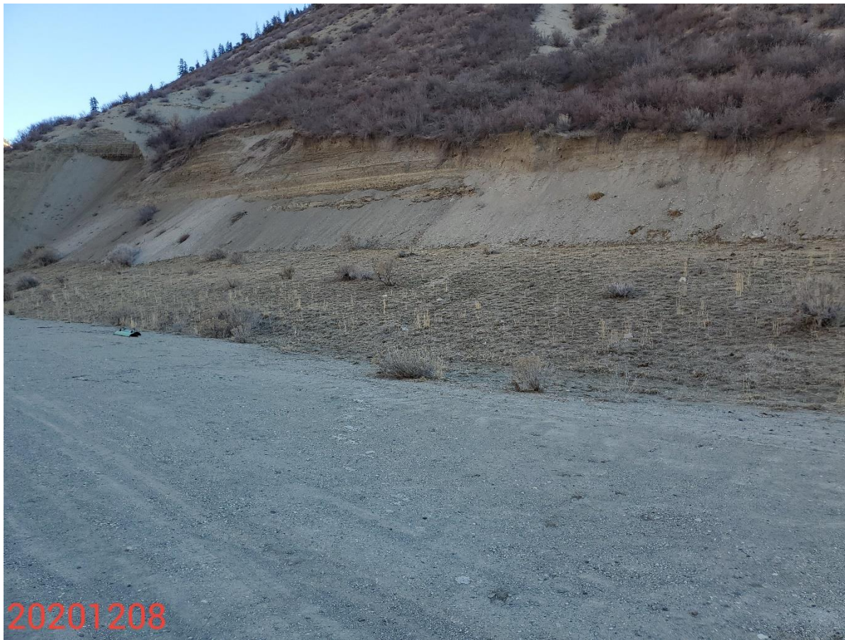
Photo 2: Photo taken from the south end of the Location, facing northeast. Photo shows BMPs to stabilize and protect cut slopes remain missing or insufficient.
