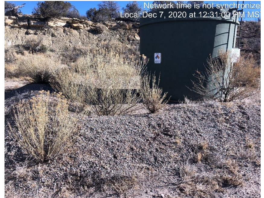
Photo #2414 Vegetation growing on secondary containment.
