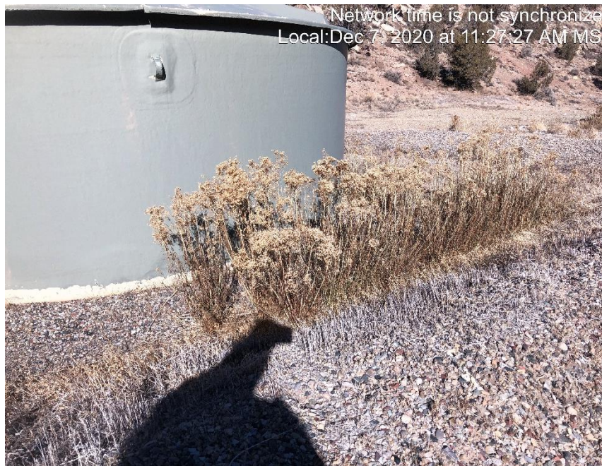
Photo #2407 Secondary containment not adequate weeds and debris inside tank containment.
