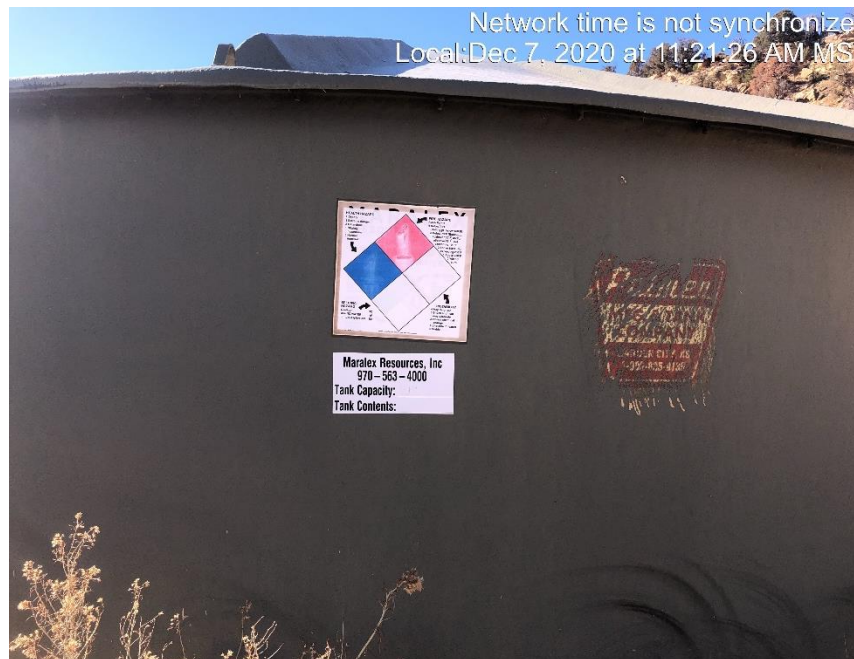
Photo #2404 Tank label weathered and not legible.
