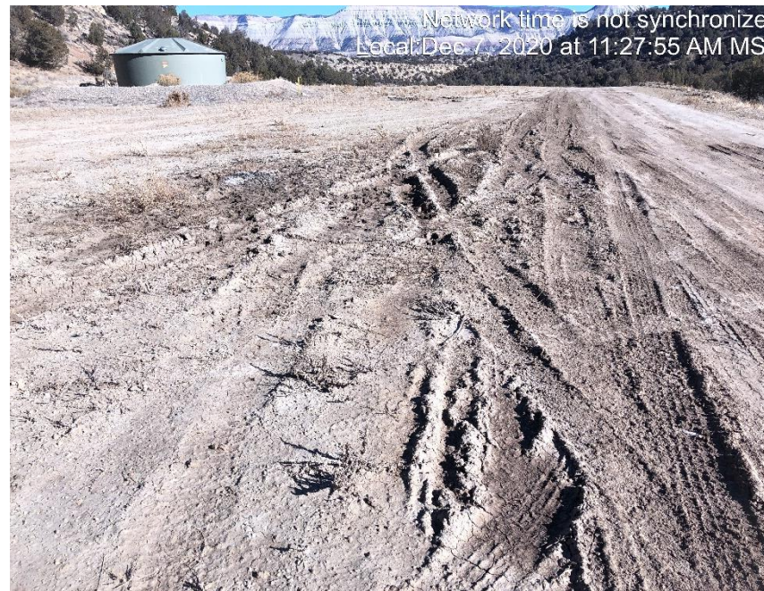
Photo #2408 Rutting occurring on location due to lack of stabilization.
