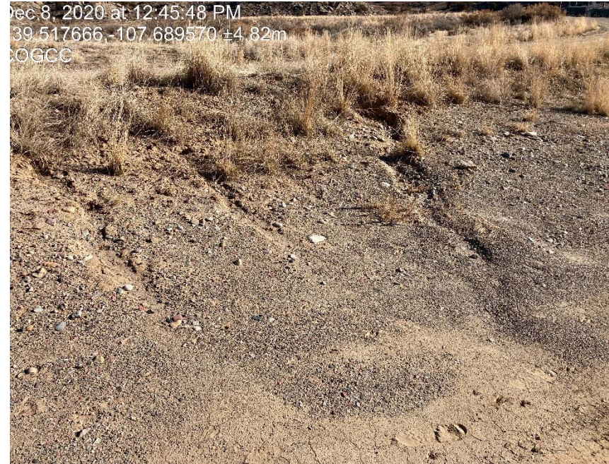
Lack of stabilization/erosion is evident (riling)
