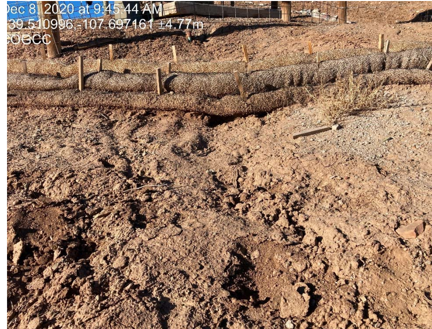
Lack of stabilization/erosion is under mining waddles
