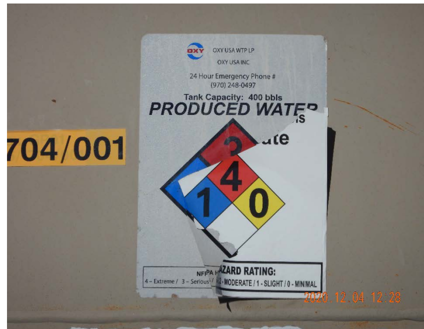
Photo #4 – Damaged NFPA placard on steel AST.
