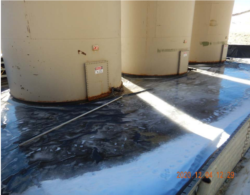
Photo #5 – Accumulation of ice inside of secondary containment area.
