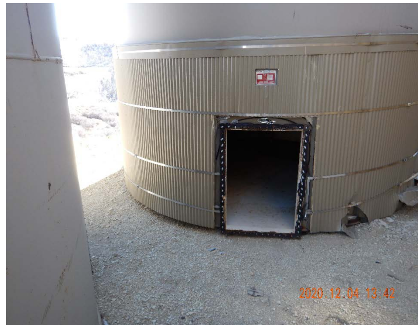
Photo #8 – Tank in tank storage area lacks access panel cover.
