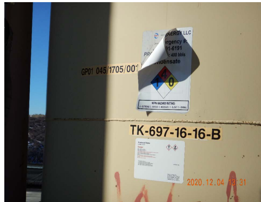
Photo #4 - NFPA placard peeling from tank (2).
