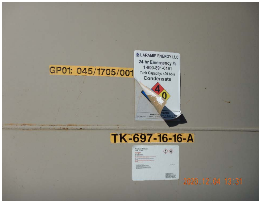
Photo #3 – NFPA placard peeling from tank (1).
