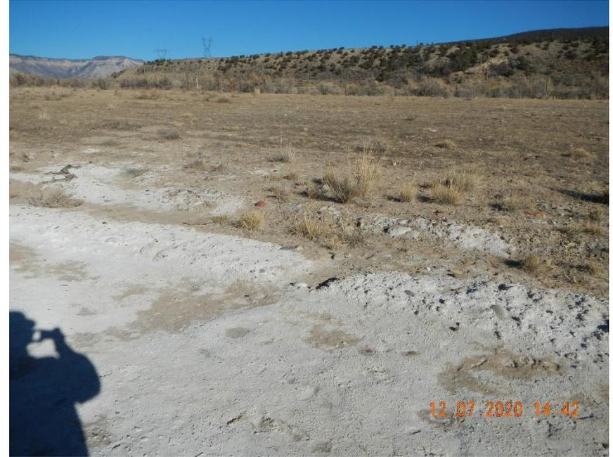
**Berm around location is breached in several areas. Ditch around location not maintained.**
