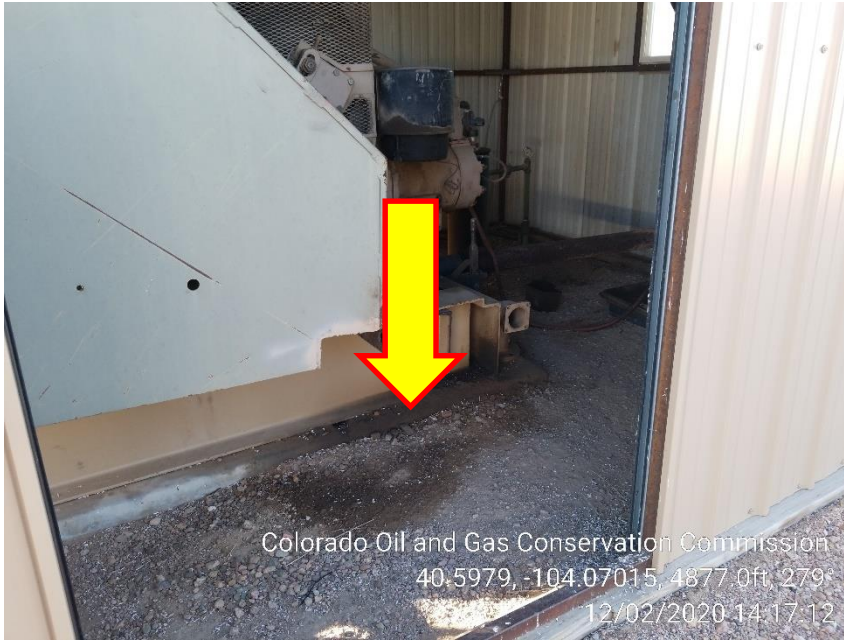
Photo 5 – Stained Soil at Gas Engine
