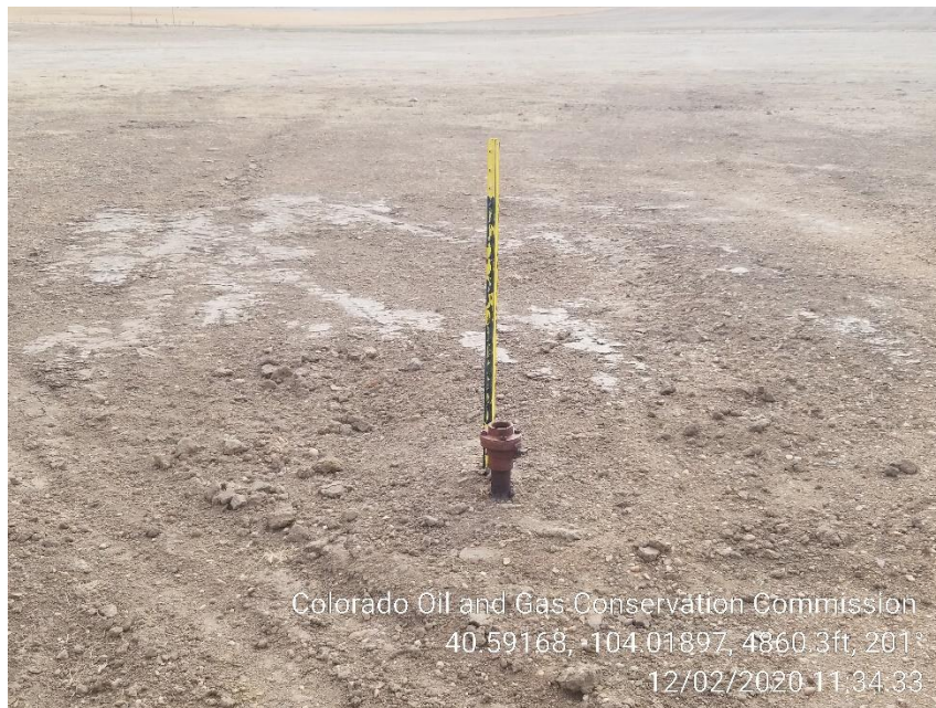
Photo 1 – Well Plugged and Abandoned, Flowline Riser remains
