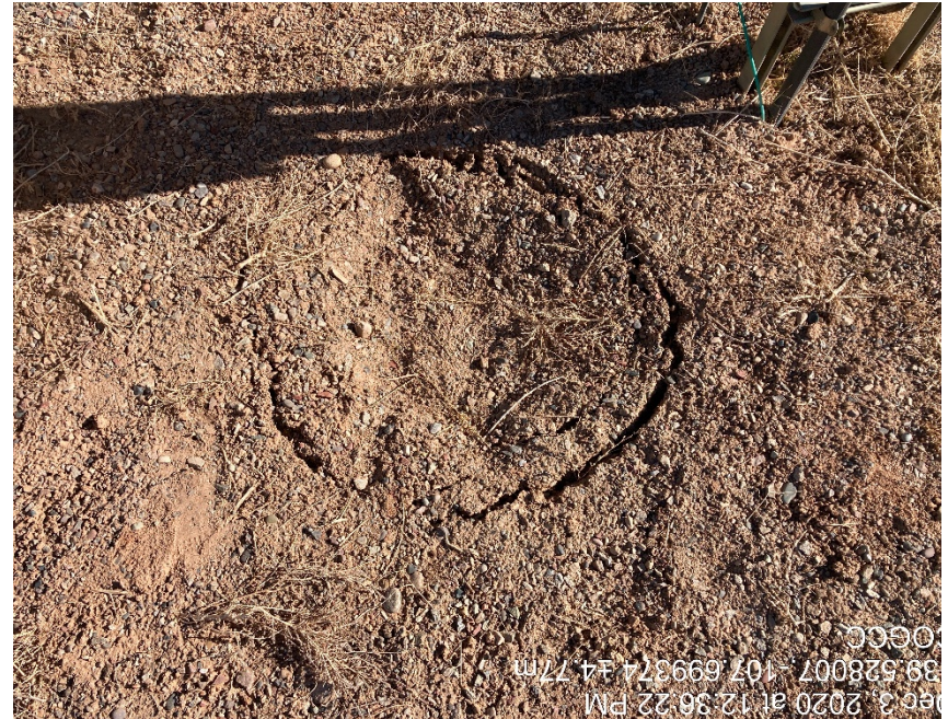
Lack of stabilization next to tank battery
