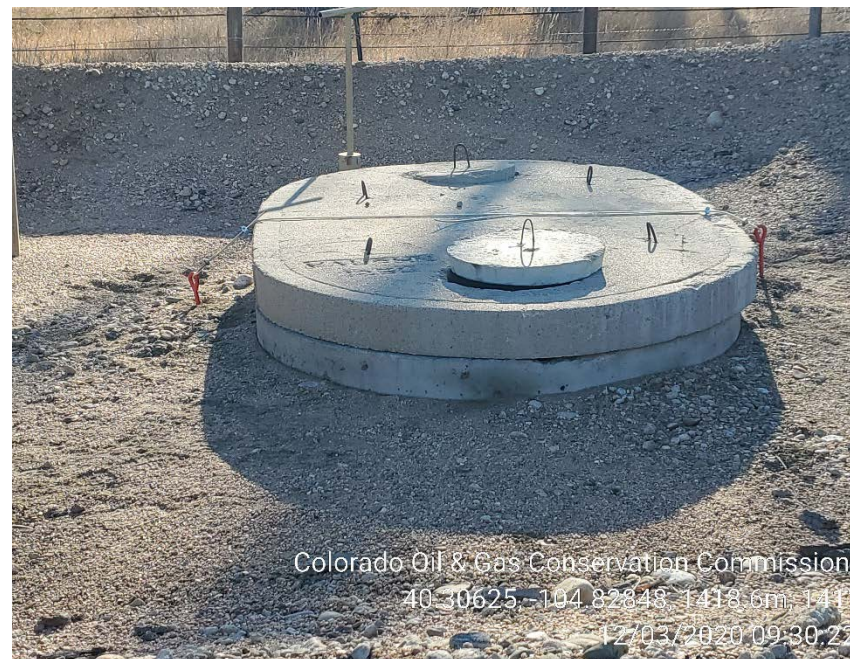
Produced water vault anchoring on 12/3/2020
