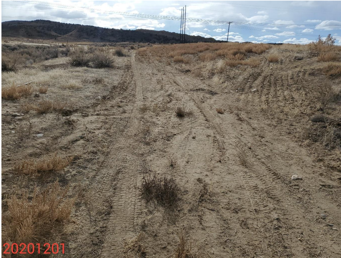
Photo 6: Photo taken from the access road north of the Location, facing south. Photo shows that a portion of the access road between the turn-off and the Location has not been reclaimed per corrective actions and rules. Vehicle travel over the reclamation area evident; Continued vehicle use is not conducive to reclamation.
