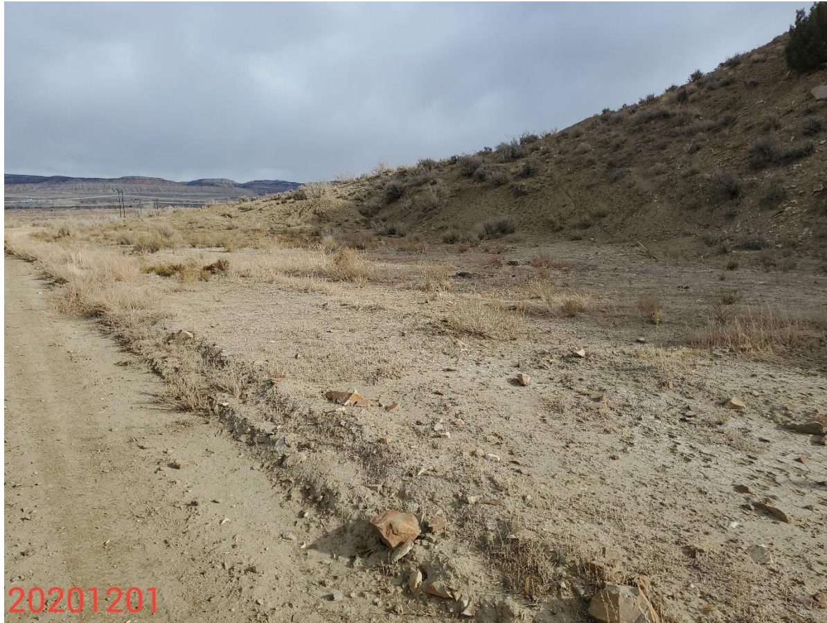
Photo 1: Photo taken from the west end of the Location, facing north. Photos 1-4 provide an overview of the Location from north, northeast, southeast to south. Photos show Location remains predominantly bare/exposed soils. Cut-slopes not reclaimed/revegetated or stabilized.
