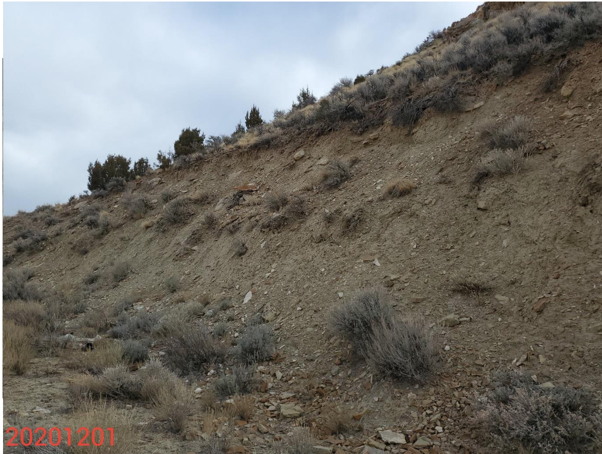
Photo 7: Photo taken from the east end of the Location, facing northeast. Photo shows cut-slopes have not reclaimed/revegetated or stabilized.
