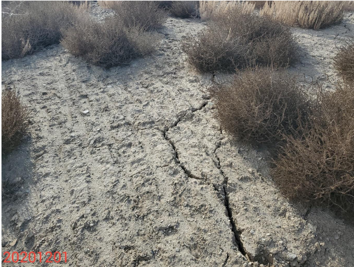
Photo 3: Photo taken from the Location. Previous inspections observed that Operator has installed tracking on the slopes of the pad; Vertical tracking is a temporary erosion control with an approximate lifespan of 2 weeks to a month, and should be used in conjunction with other BMPs. Photo shows that no additional BMPs have been used in conjunction with the vertical tracking, and cracking/rilling now evident.
