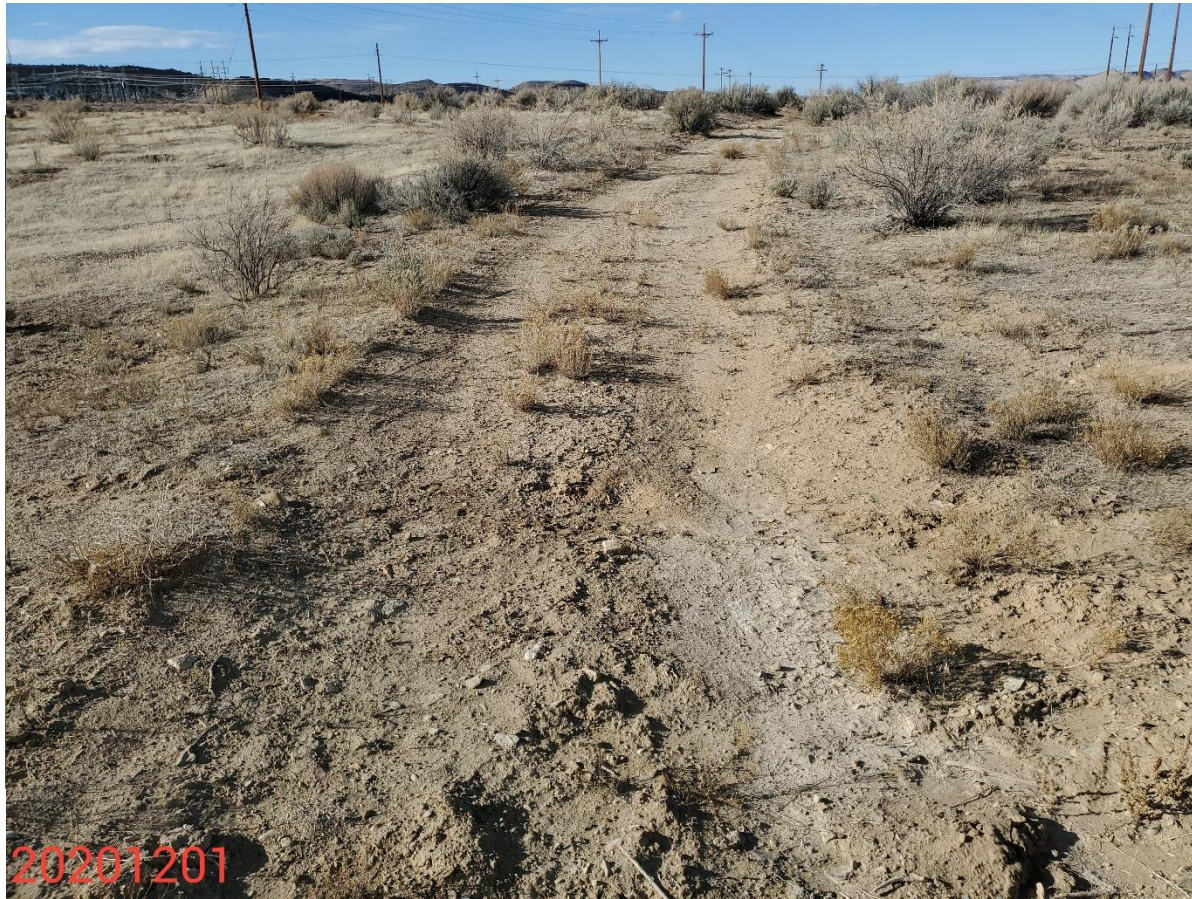
Photo 7: Photo shows access road west of the Location. Reclamation activities pursuant to Rule 1004.a has not been conducted including compaction alleviation.
