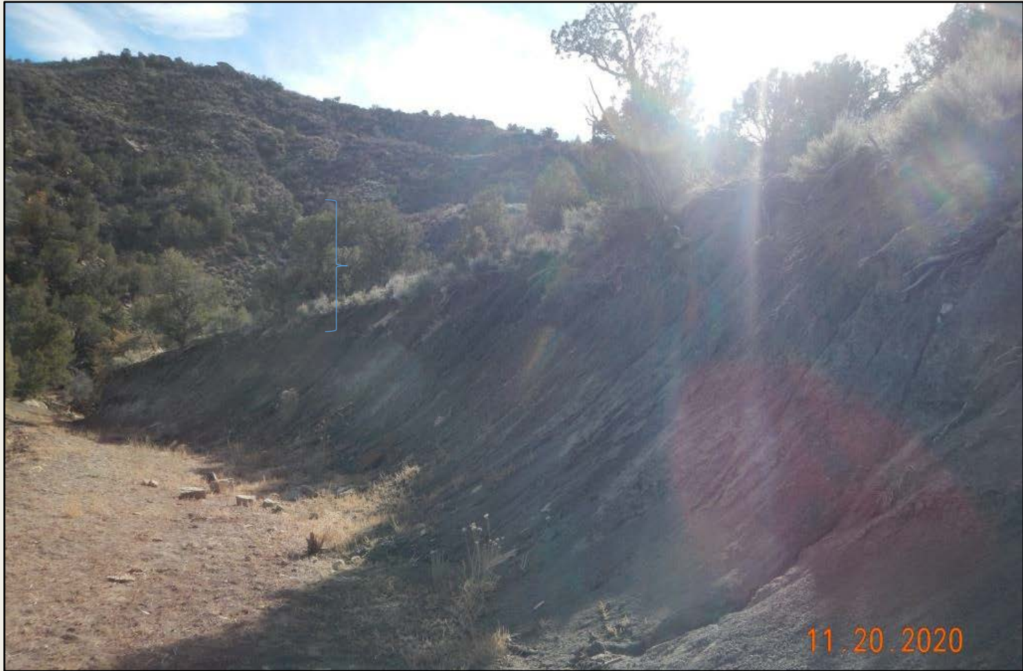
Photo 2. View of eroding cut-slope within the southern project area. Erosional channels, exposed roots, and sediment plumes observed.
