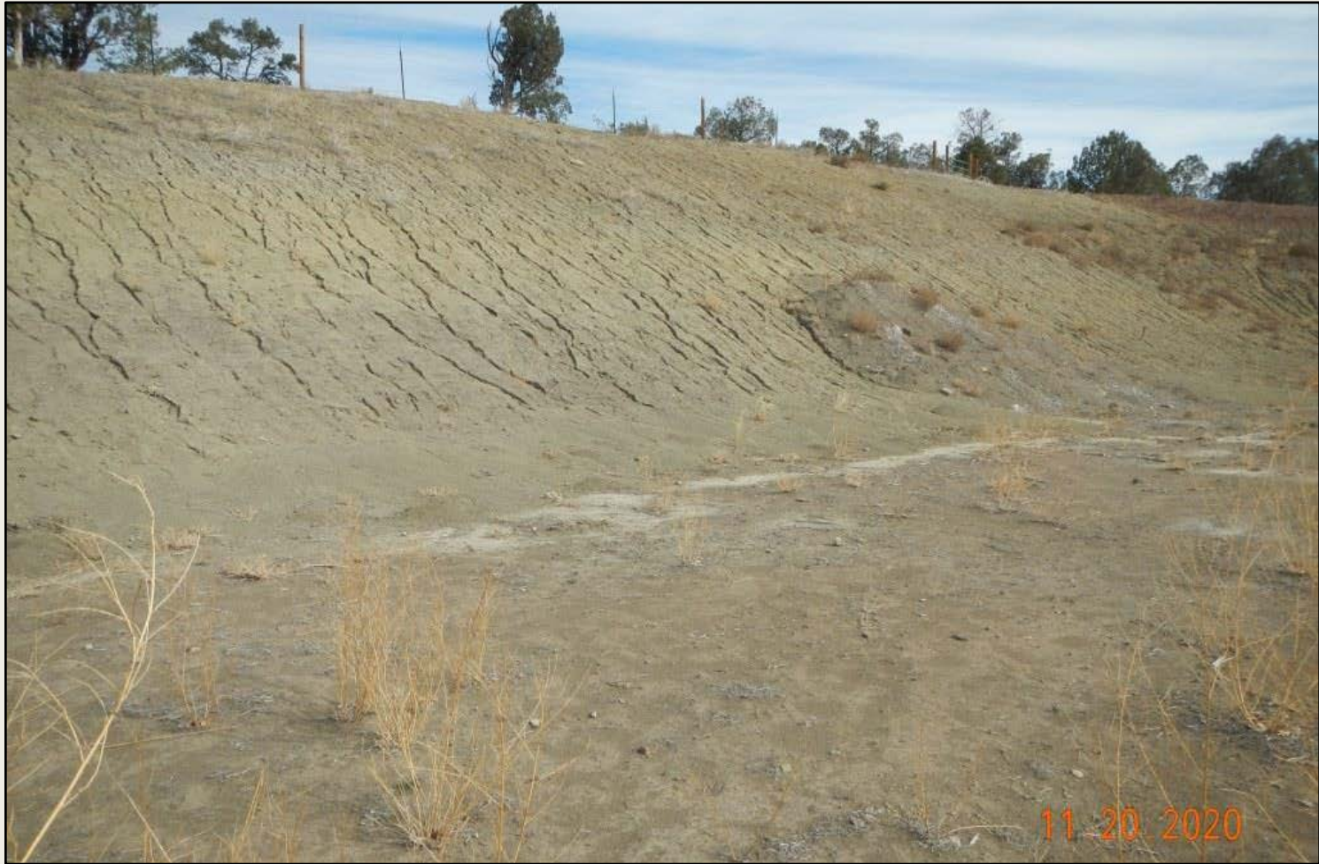
Photo 3. View of the northern project area from the northeastern corner facing westward. Cut slope is largely bare and rapidly eroding.
